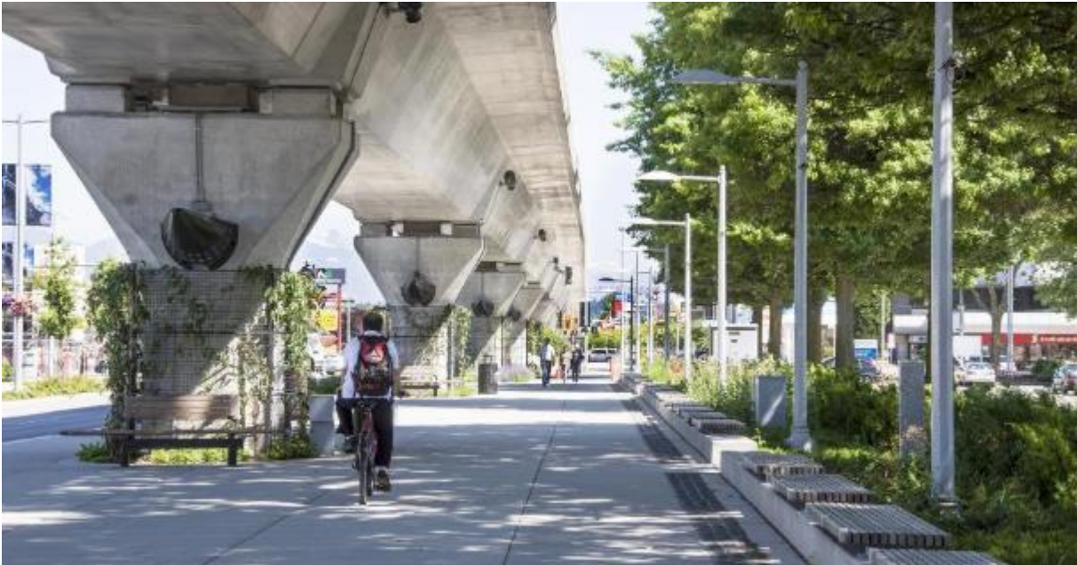
Opportunities exist to install planting beds or vertical vegetative screens around the SkyTrain's guideway columns.
