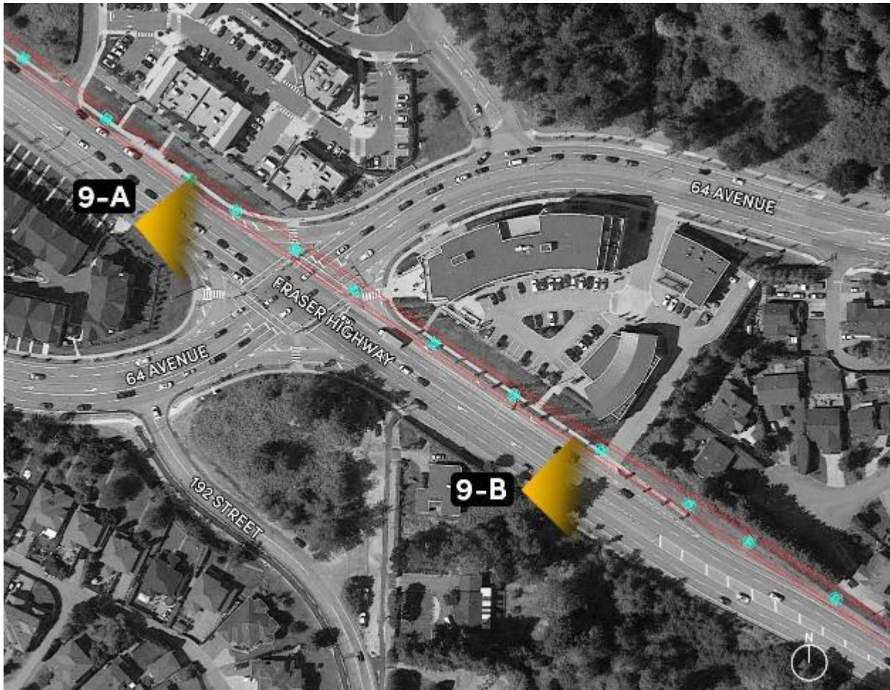
Figure 16-30 Location 9: Guideway at Fraser Highway near 64 Avenue Showing Viewpoint
