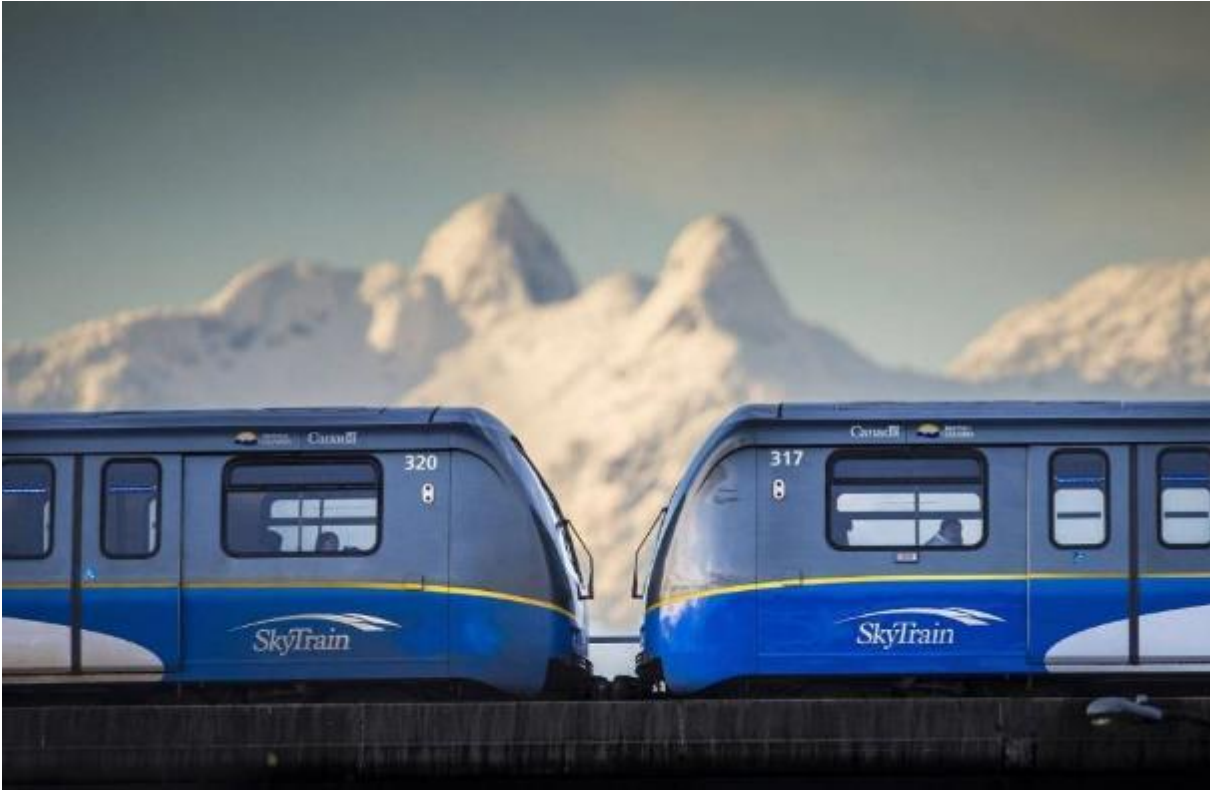
The SkyTrain guideway provides unobstructed views of the North Shore mountains.
