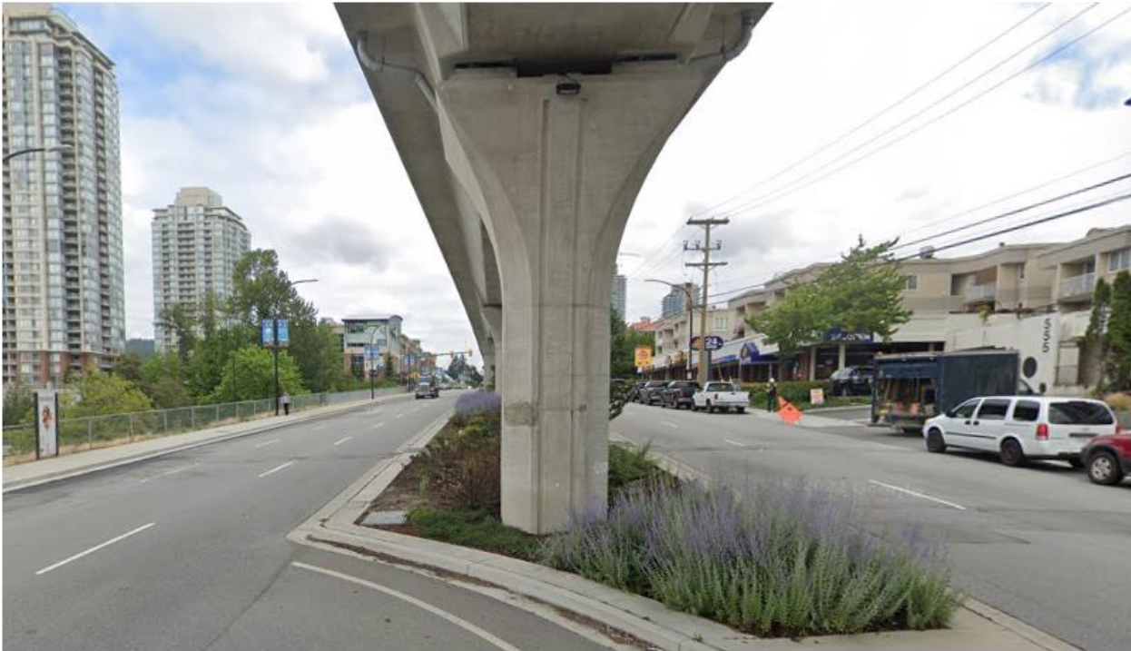
Figure 2-10 Typical Guideway Column Design
