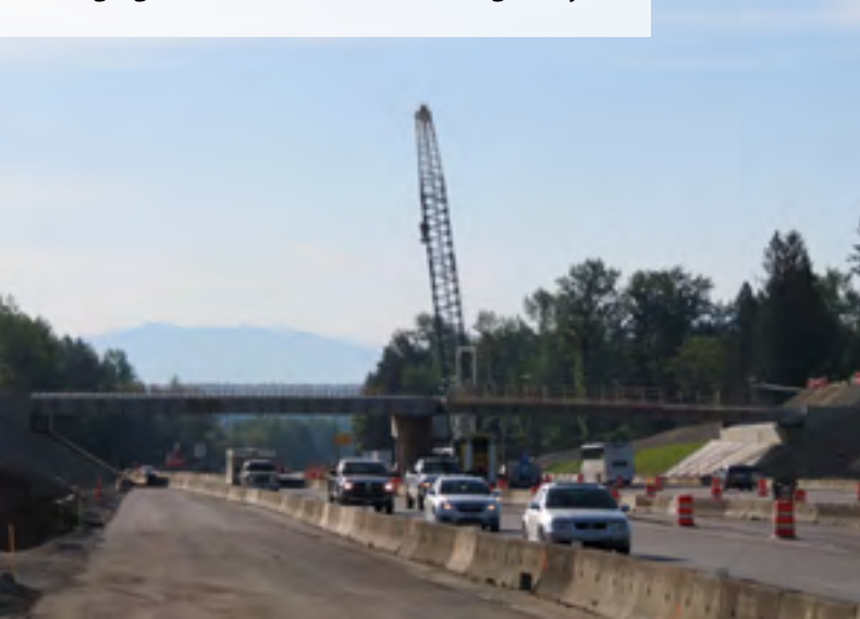
Bridge girder installation over Highway 1
