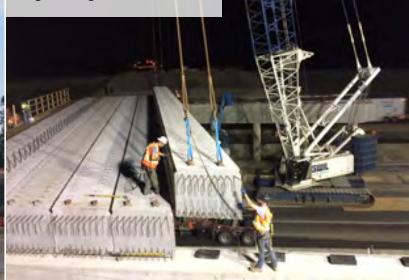
Nighttime girder installation
