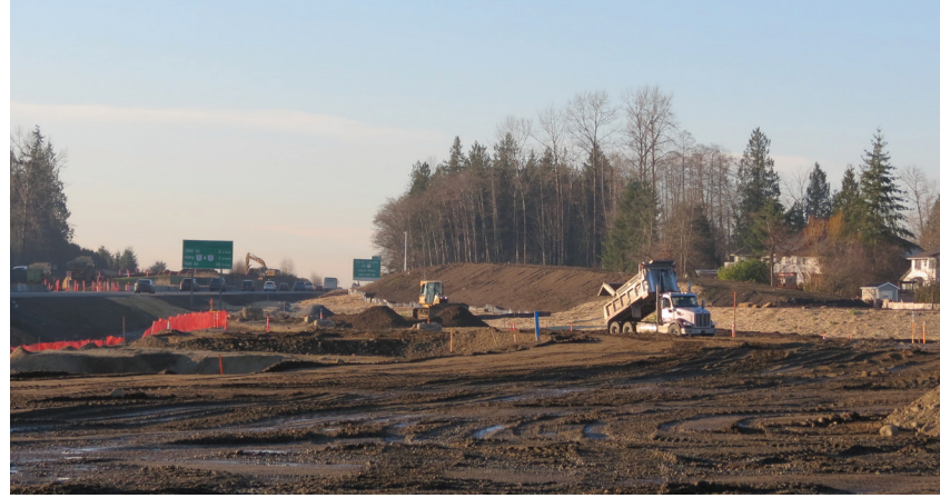
Site grading and fill material collection for interchange ramps and structure
