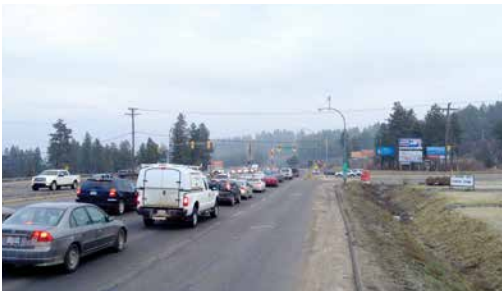
Highway 97 approaching the existing Boucherie Road intersection
