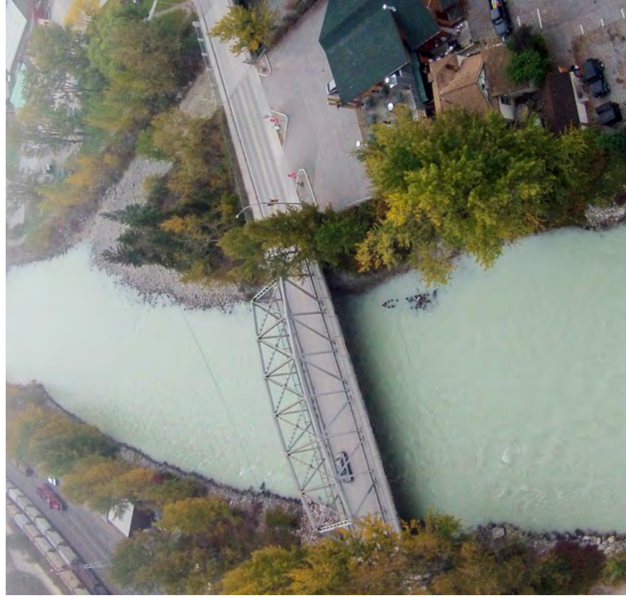
Aerial view of existing Kicking Horse River Bridges 1 & 2
