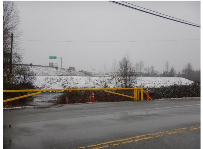
River Road Looking at Preload. Taken Jan 31, 2020
