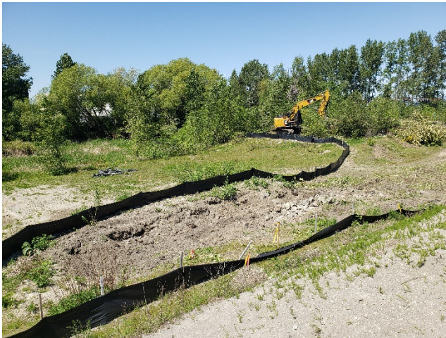
Segment 1 clearing work. Taken May 14, 2020
