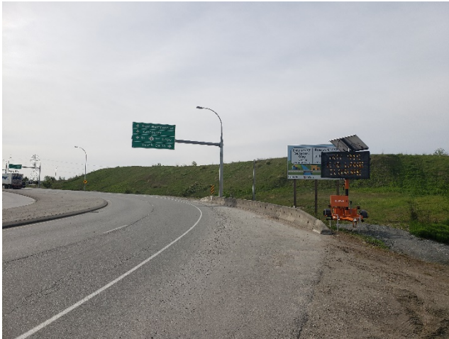
Hwy 91C EB lane closure. Taken May 4, 2020
