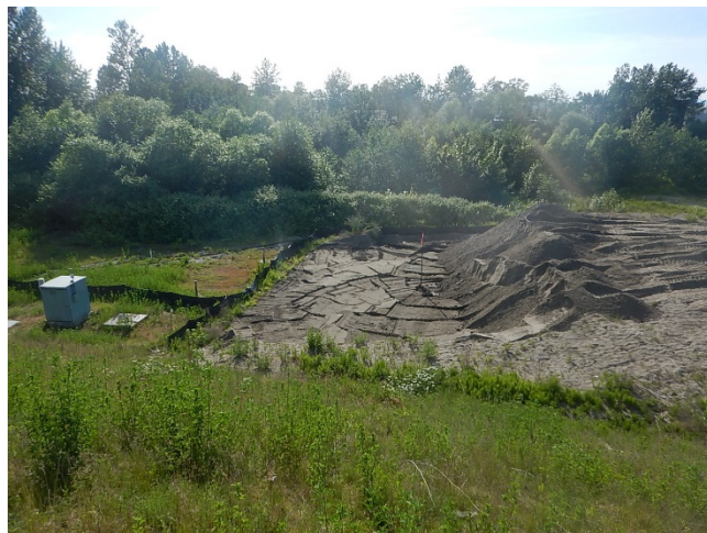
Segment 1 fill placement. Taken May 28, 2020
