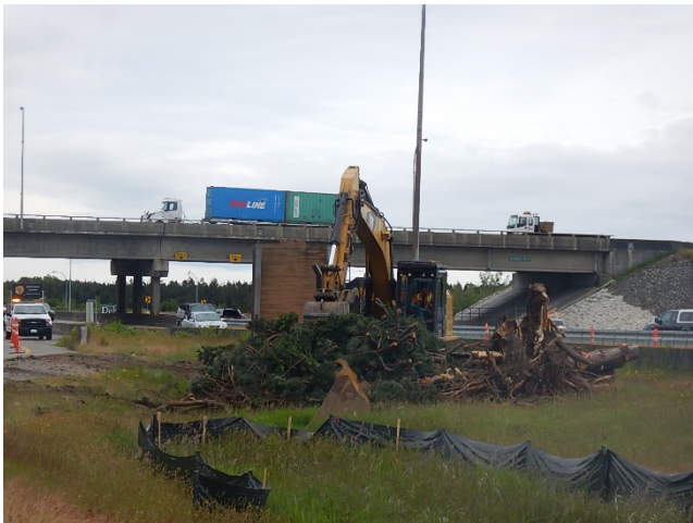
Segment 4 clearing work. Taken June 11, 2020
