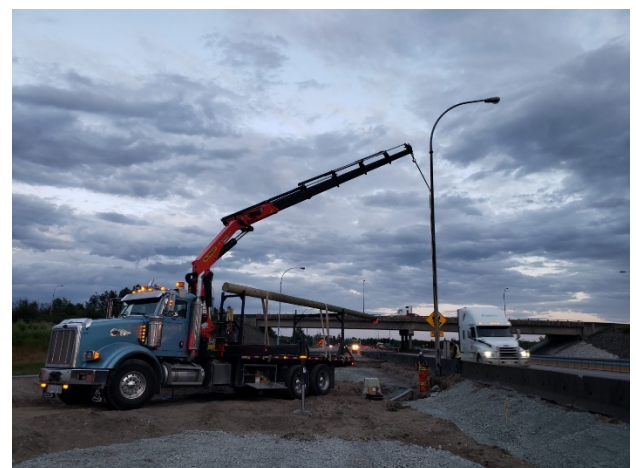
Pole relocation. Taken June 29, 2020
