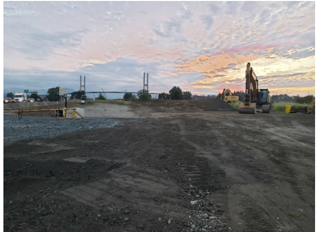
S2: Hwy 91C/17 (Sunbury) Interchange – Access/egress points created. Taken July 16, 2020
