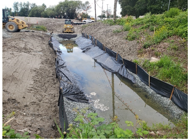
S1: River Road West Roundabout – Ditch protection in place. Taken July 7, 2020
