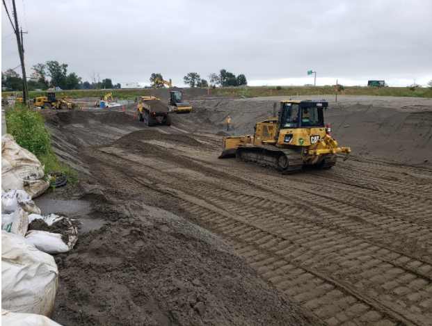
S1: River Road West Roundabout – Preload/embankment fill placement underway. Taken July 2, 2020
