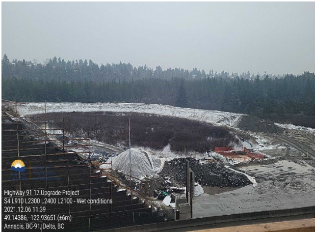
S4: Wet conditions on site. Taken December 6, 2021
