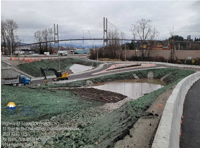
S1: River Road east roundabout - hydroseeded slopes. Taken December 1, 2021
