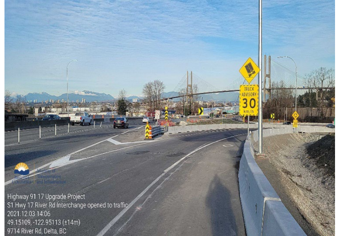
S1: Hwy 17 River Road Interchange opened to traffic. Taken December 3, 2021
