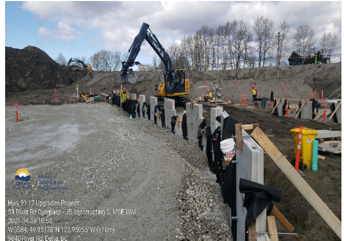
S1: River Road structure - S. MSE wall construction. Taken April 8, 2021
