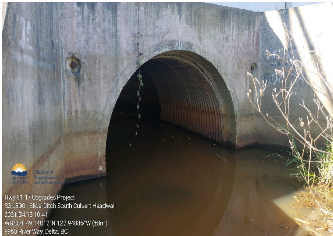
S3: Silda Ditch south culvert headwall. Taken April 13, 2021
