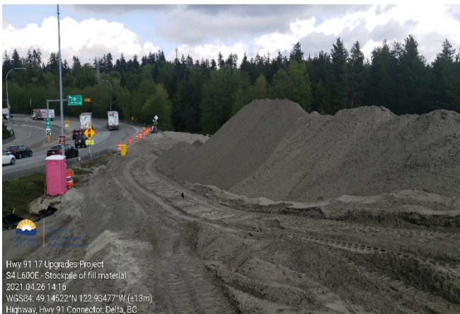
S4: Hwy 91 east side stockpile of fill material. Taken April 26, 2021
