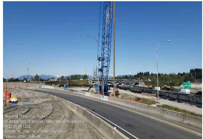
S4: Nordel Way structure crane move. Taken April 19, 2021
