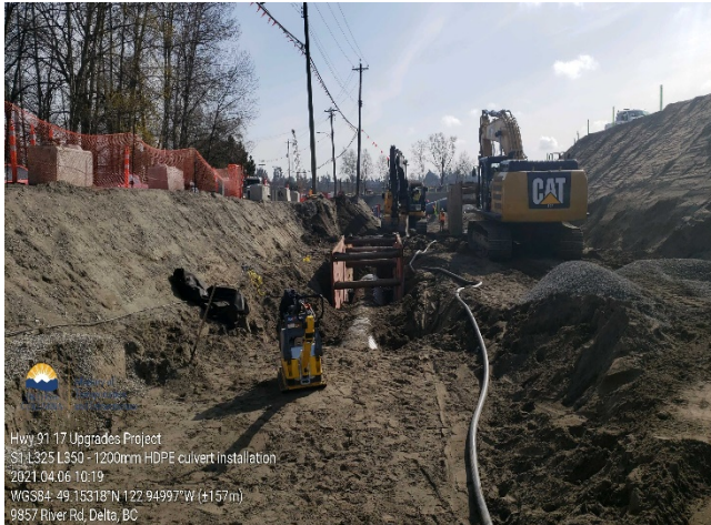
S3: 1200mm HDPE culvert installation. Taken April 6, 2021
