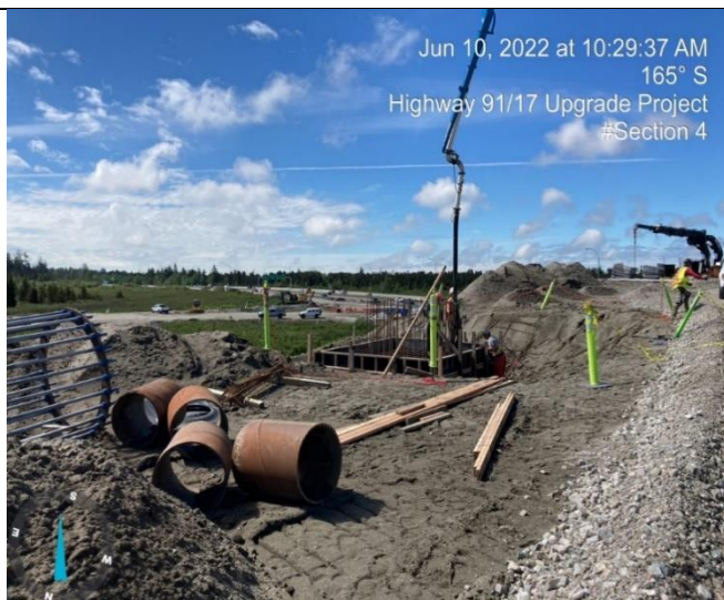
Photo 67: L2300 (G). Concrete being poured into framework for guide sign.
