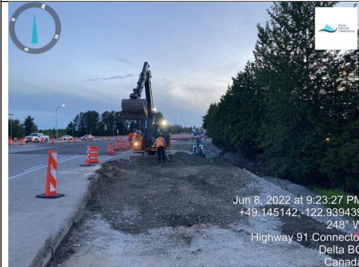
Photo 59: L2250 (I). Gravel placement.
