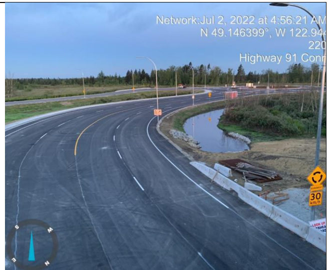
Photo 46: L1150 (F). Paving complete.
