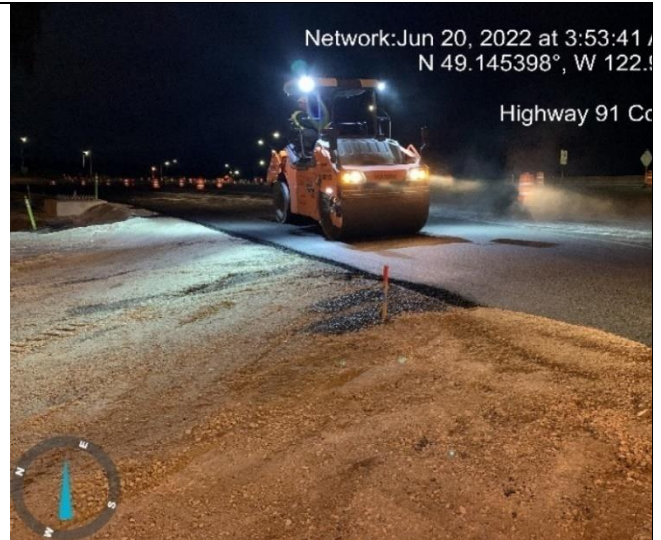
Photo 64: L2250 (I). Paved the remaining base lift.
