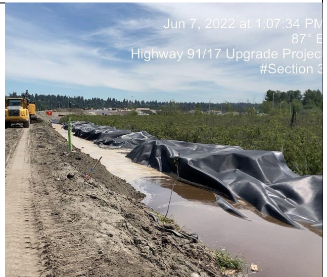
Photo 26: L1170 (F). Bog liner install.
