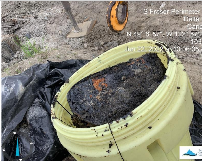
Photo 89: Hazardous waste material from Sunbury Mounds contained for removal from site by Secure Energy.
