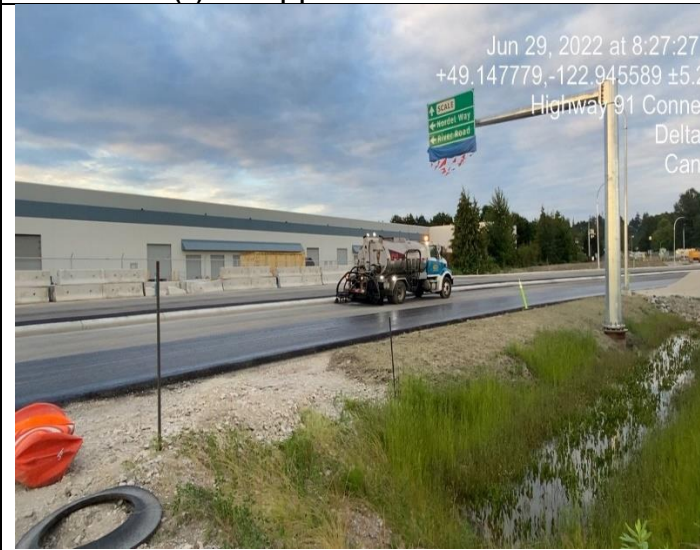
Photo 53: L1130 (H). Tack being applied prior to asphalt placement.
