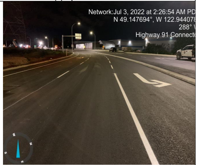
Photo 54: L1300 (H). Night shift paving complete.
