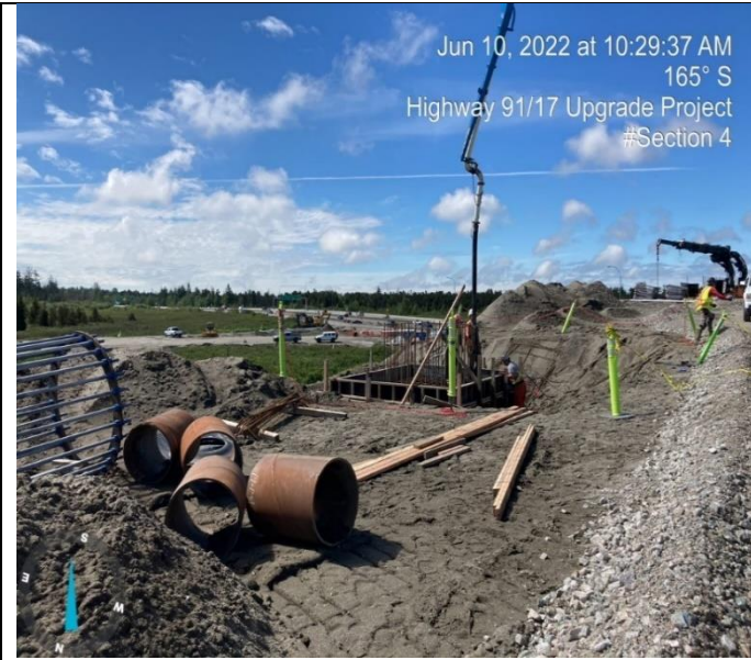
Photo 69: L2300 (G). Guide sign concrete pour into formwork.
