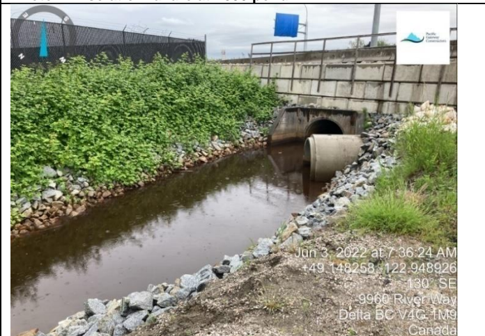
Photo 79: Culvert discharge location in Silda Ditch, 3 June 2022 at 07:46 (30.92 NTU)
