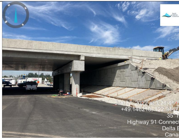
Photo 19: L500 (E). S3 bridge south side.
