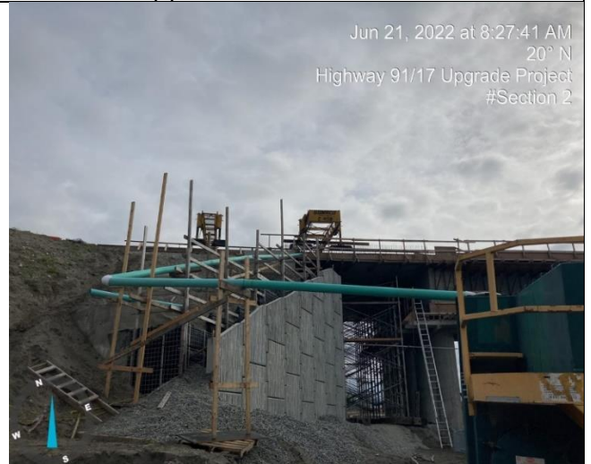
Photo 18: L500 (S2 Bridge). Curing water holding tank system installation.
