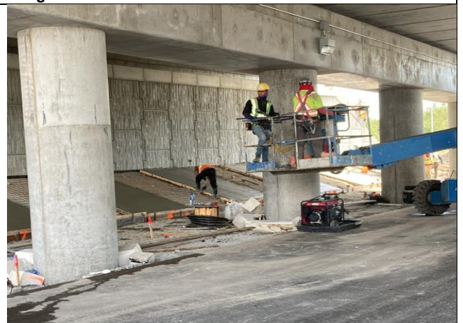
Photo 42: L1150 (F). S3 bridge spillway concrete pour.
