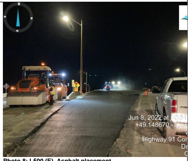
Photo 8: L500 (E). Asphalt placement.
