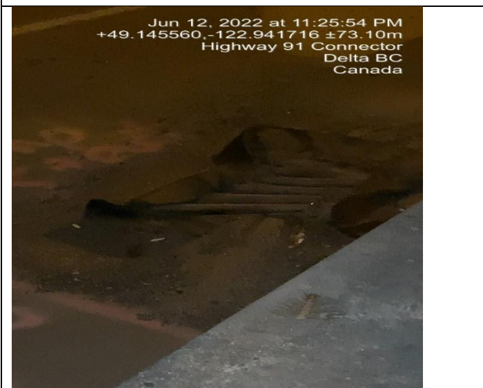
Photo 61: L500 (I). Catch basin inserts installed for paving activity.
