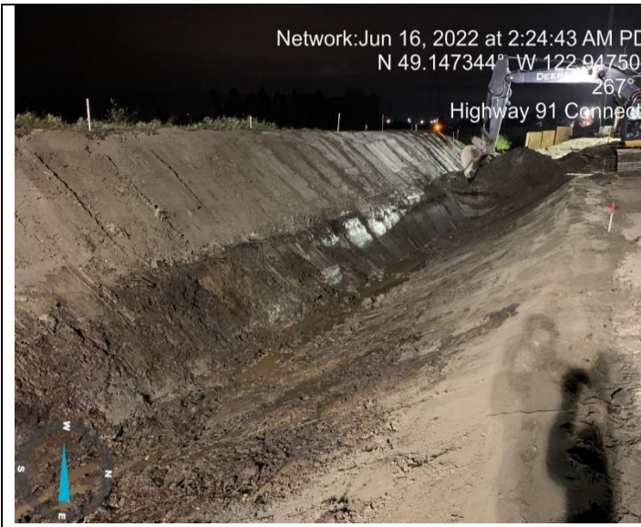
Photo 33: L1170 (F). Cutting ditches.
