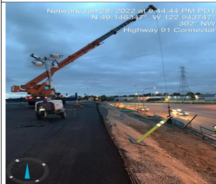
Photo 43: L1150 (F). Removed lock blocks from wall.
