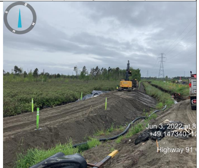
Photo 24: L1170 (F). Burns Bog berm construction.
