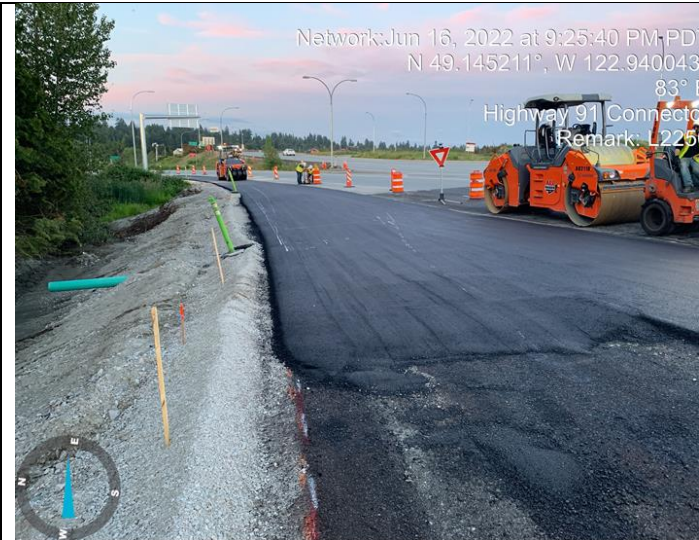
Photo 63: L2250 (I). Paved the road widened area
