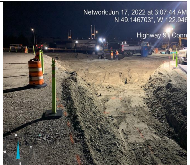
Photo 34: L1170/L1160 (F). Excavation for gore
