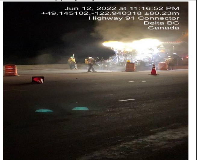
Photo 60: L500 (I). All Roads asphalt placement.
