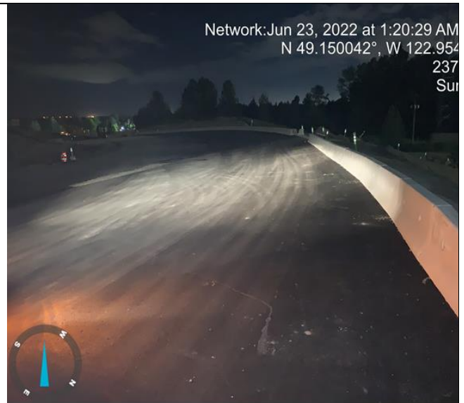
Photo 16: L400 (E). New barriers installed.
