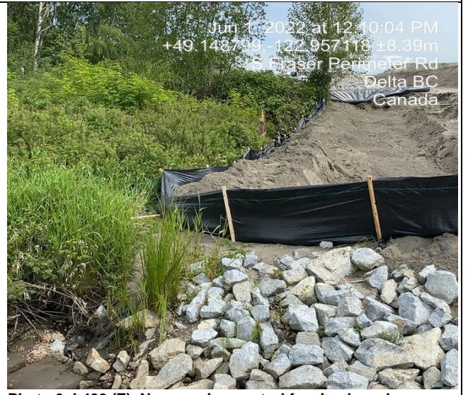
Photo 6: L400 (E). New erosion control fencing keyed.
