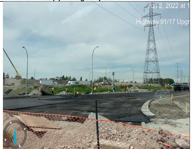
Photo 48: L1300 (H). Placing asphalt geogrid.
