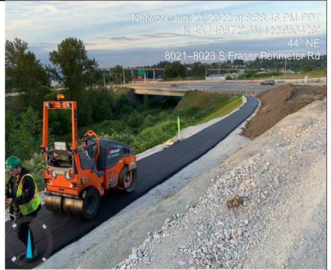
Photo 12: L550 (E). Bike path asphalt placement.
