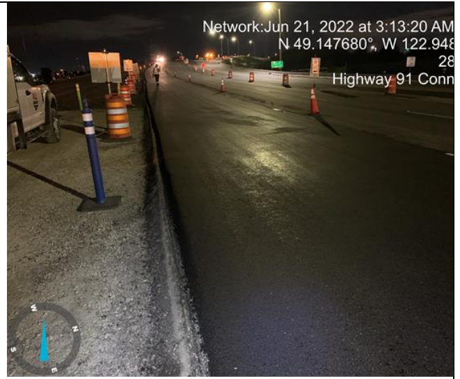
Photo 22: L500 (E/H). Leveling course asphalt placement.
