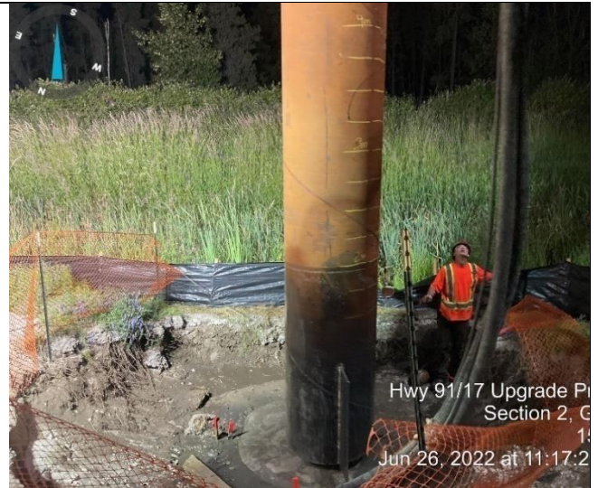
Photo 4: L100 (A). Guide sign piling.
