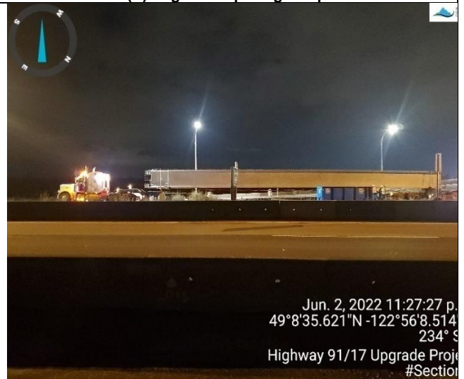
Photo 56: L2200 (I). S4 bridge girder receipt.
