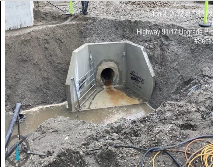
Photo 57: L2250 (I). Head wall installed.
