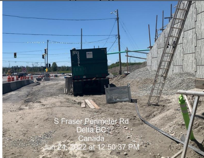
Photo 17: L500 (E). S2 bridge east side.
