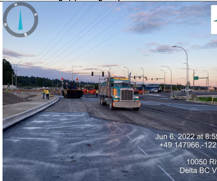
Photo 49: L1300 (H). Asphalt placement.
