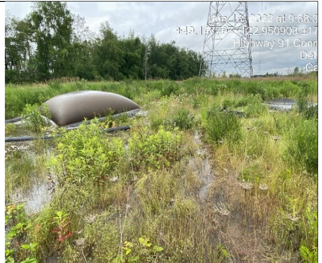
Photo 10: L550 (E). Dewatering with 6-inch pumps.
