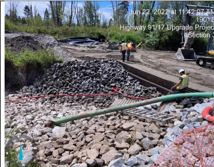
Photo 21: L1170 (E/F). Bog berm MSE wall progress.
