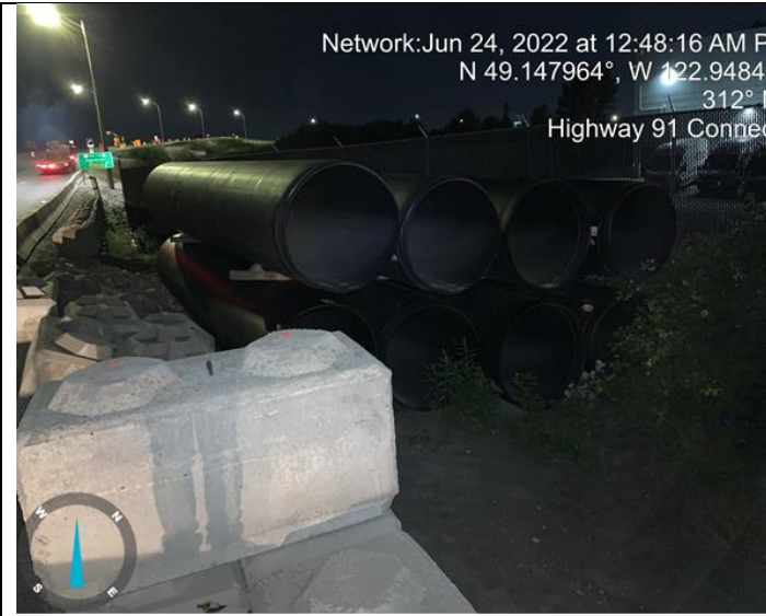
Photo 51: L500 (H). HDPE pipes moved to WB 91.
