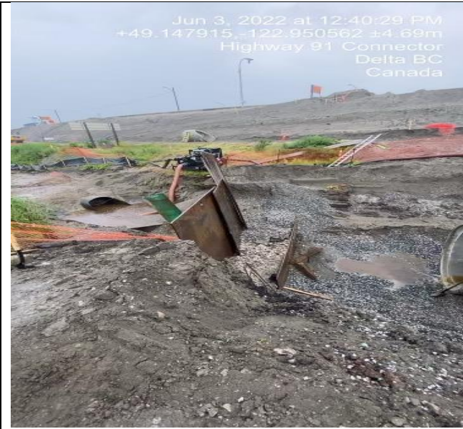
Photo 81: Re-established isolation at L500 pond.
