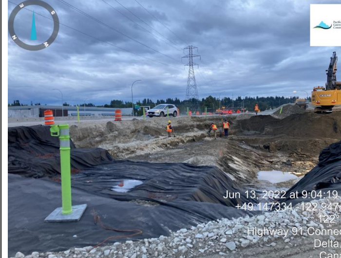
Photo 29: L1160 (F). Excavation for cellular concrete fill by pumice.
