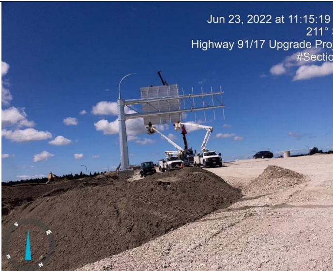
Photo 73: L2300 (G). Installing a guide sign.
