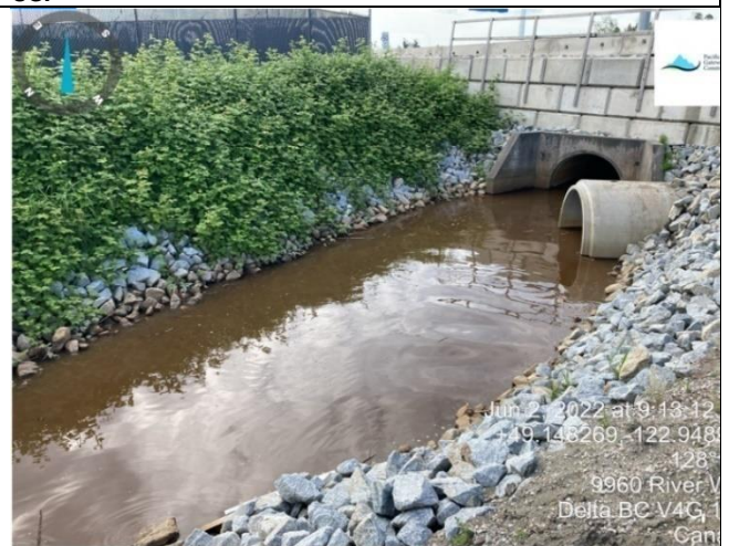
Photo 78: Culvert discharge location in Silda Ditch, 2 June 2022 at 09:13 (240 NTU)
