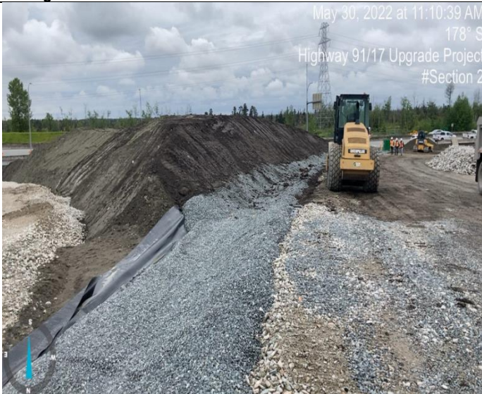
Photo 5: L400 (E). Ditching.
