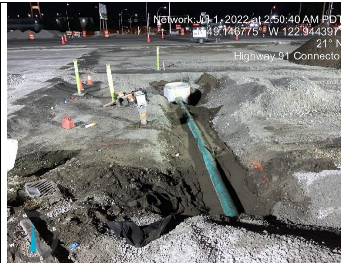
Photo 45: L500 (F). Catch basin extension work.
