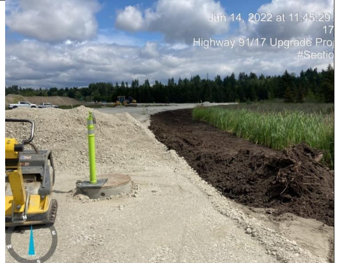
Photo 72: L2400 (G). Peat placed on top of liner
