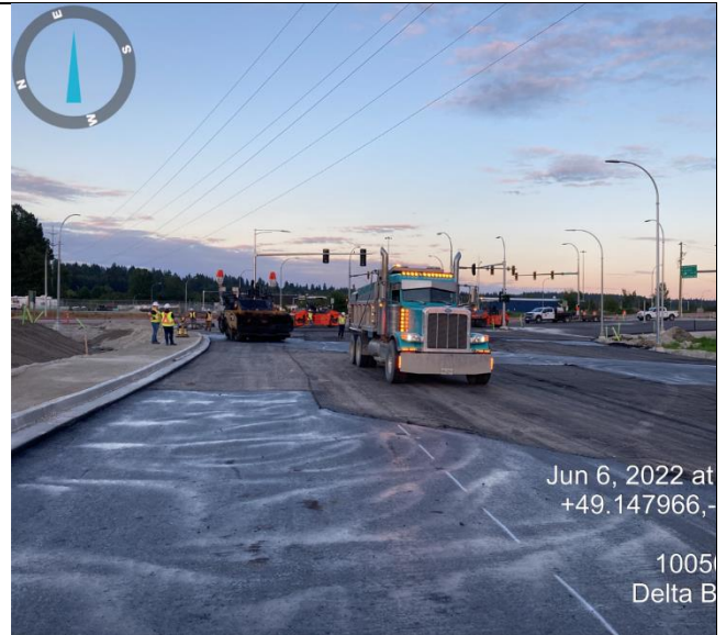
Photo 58: L1300 (H). Asphalt placement.
