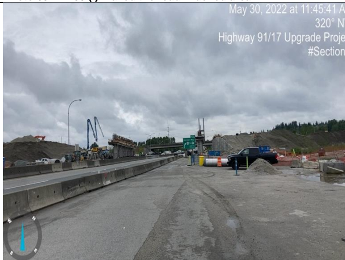
Photo 65: L600 (G). S4 bridge work and pour.
