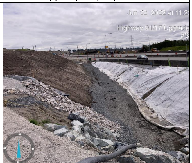
Photo 14: L400 (E). Ditch infilling.
