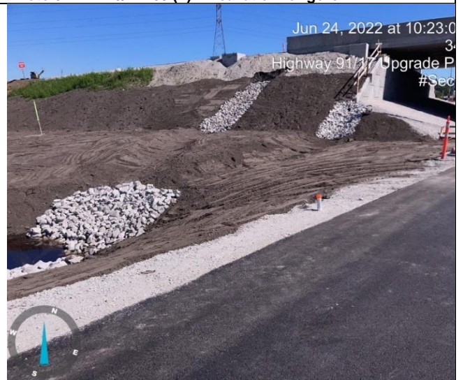
Photo 36: L1150 (F). Rip rap at S3 bridge.
