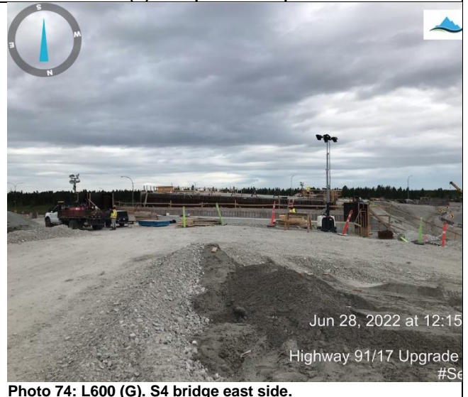
Photo 74: L600 (G). S4 bridge east side.
