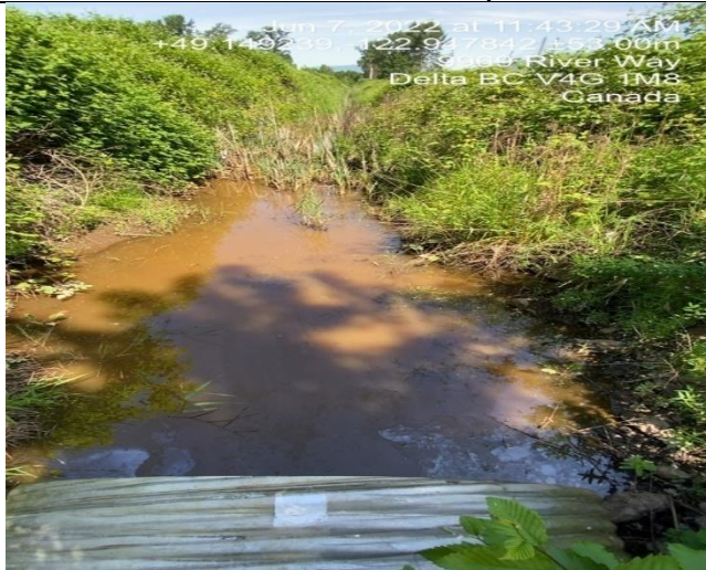
Photo 83: Low water levels and elevated turbidity at Silda midstream location.
