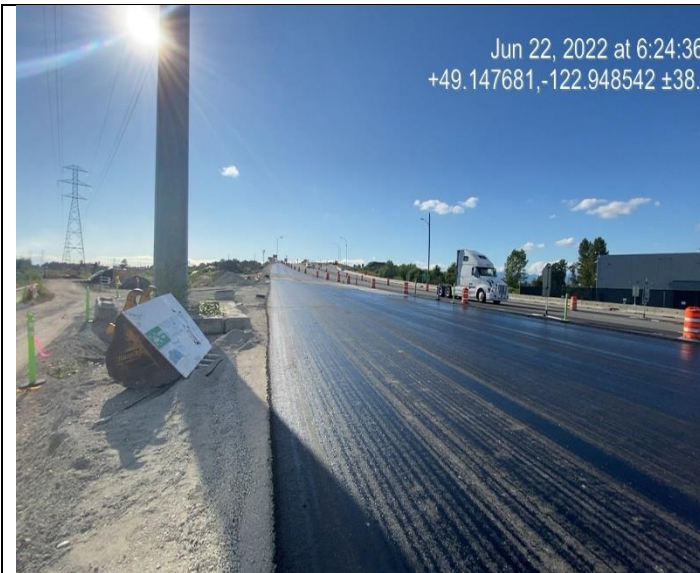
Photo 15: L1170/L500 (E). Freshly applied tack.
