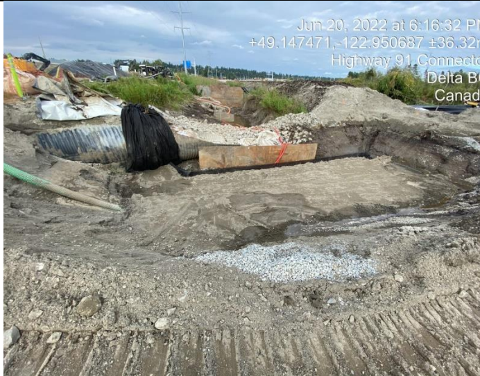
Photo 11: L550 (E). MSE wall being built.
