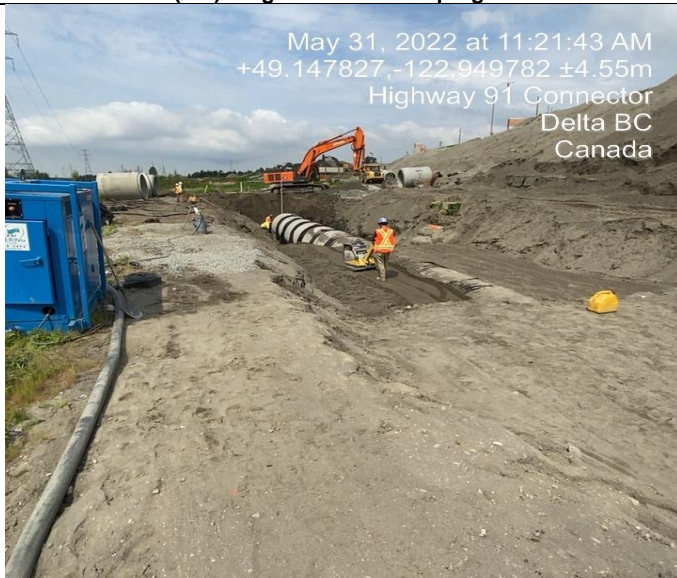
Photo 23: L1700 (F). Working on storm drain.
