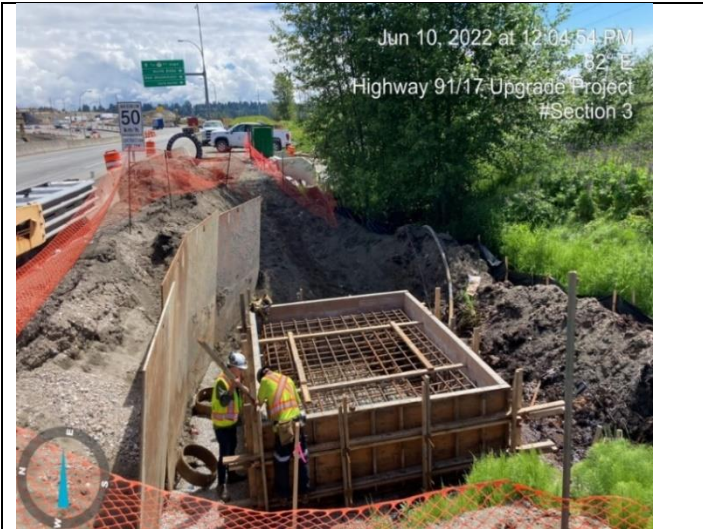
Photo 9: L550 (E). Guide sign formwork in preparation for concrete pour.
