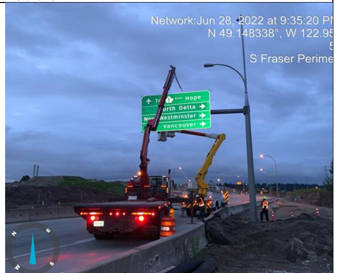
Photo 20: L550 (E). Removing existing guide signs.
