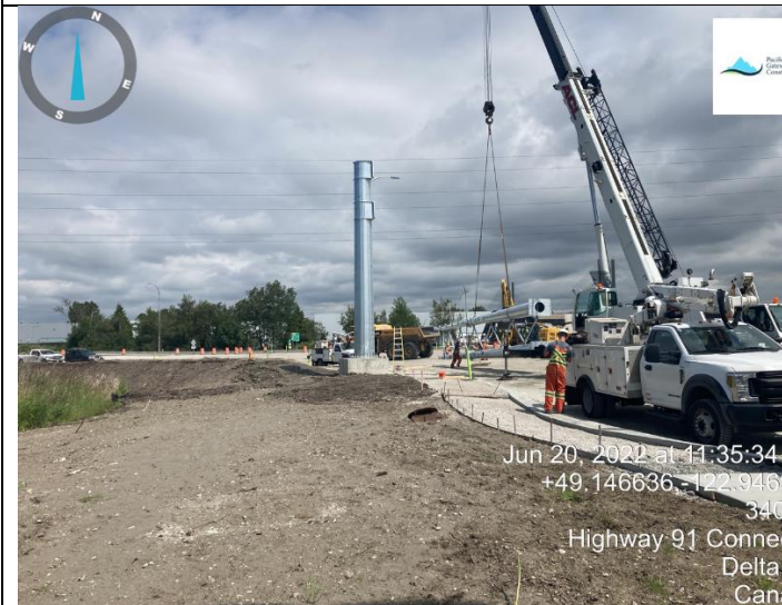
Photo 35: L1170 (F). Guide sign installation.
