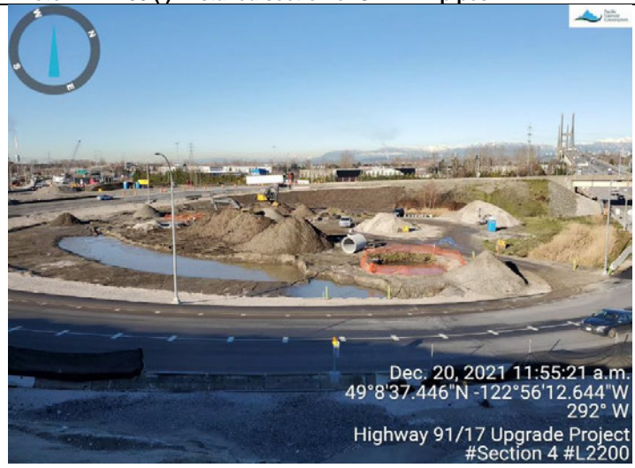
Photo 16: L2200 (I) Embankment shaping at the wetland compensation area
