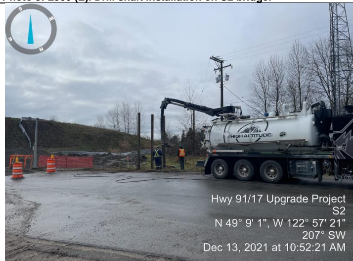
Photo 5: L500W (E). Hydrovacked utilities
