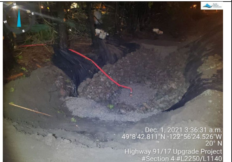
Photo 12: L2250 (I). Installed a dewatering sump.
