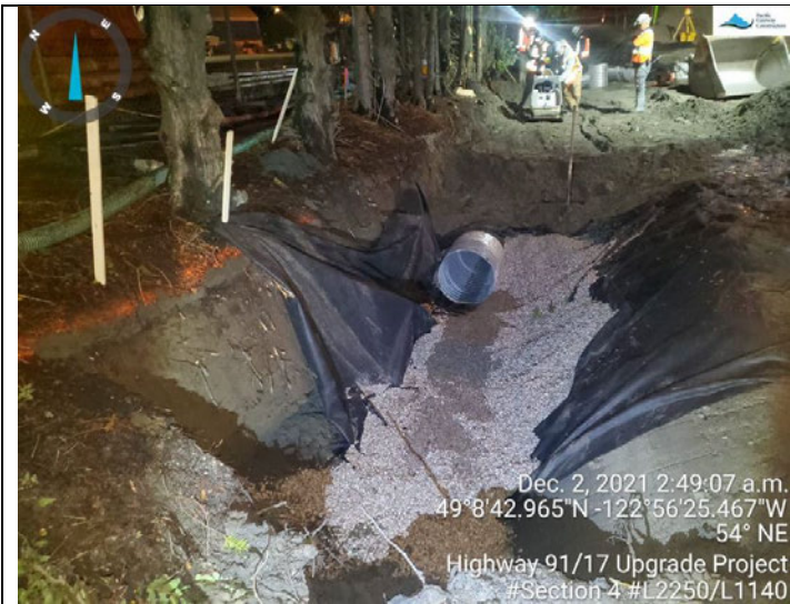
Photo 13: L2250 (I). Installed the STM 417 pipes.
