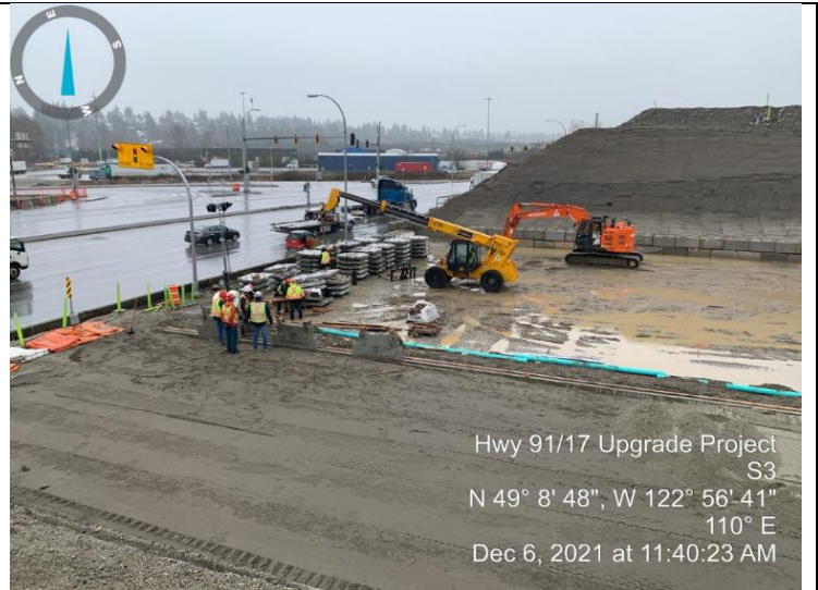
Photo 8: L500M (F). Drainpipe installation
