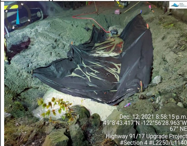
Photo 15: L2250 (I).STM 417 pipe placement
