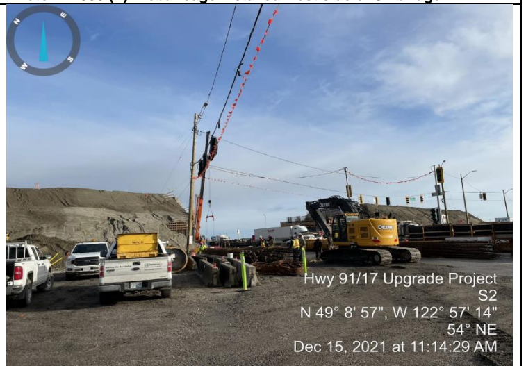
Photo 6: L500 (E). Installing columns rebar cage for S2 bridge
