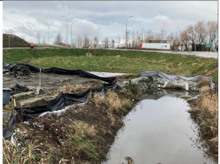
Photo 2: L325 (C) ESC fencing and erosion repairs
