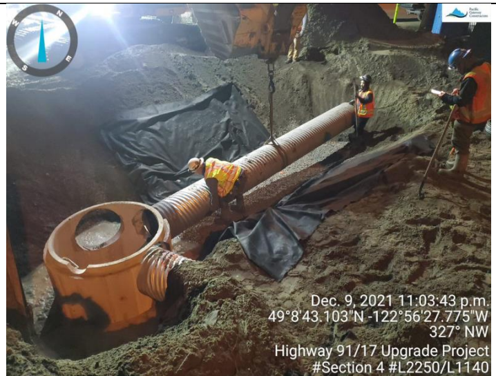
Photo 14:L2250 (I). Installed section of STM 417 pipes
