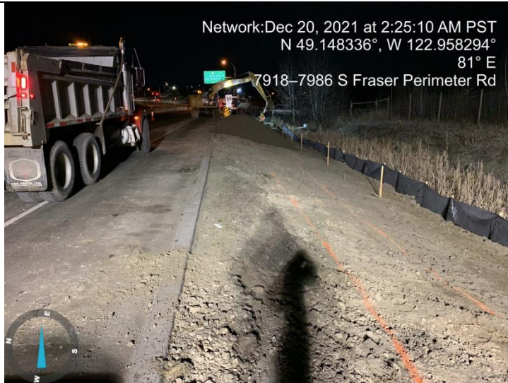
Photo 7: L500 (E). Topsoil stripping and ESC fencing placement
