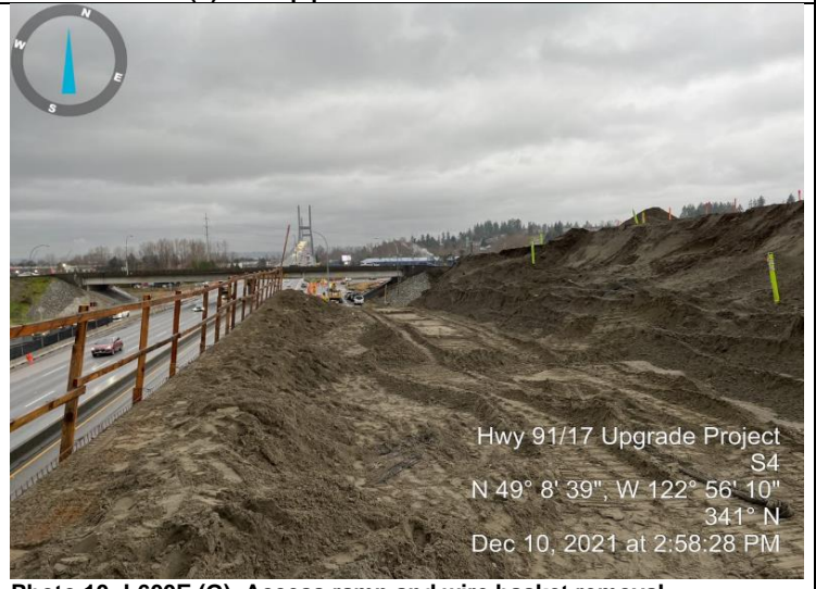
Photo 10: L600E (G). Access ramp and wire basket removal
