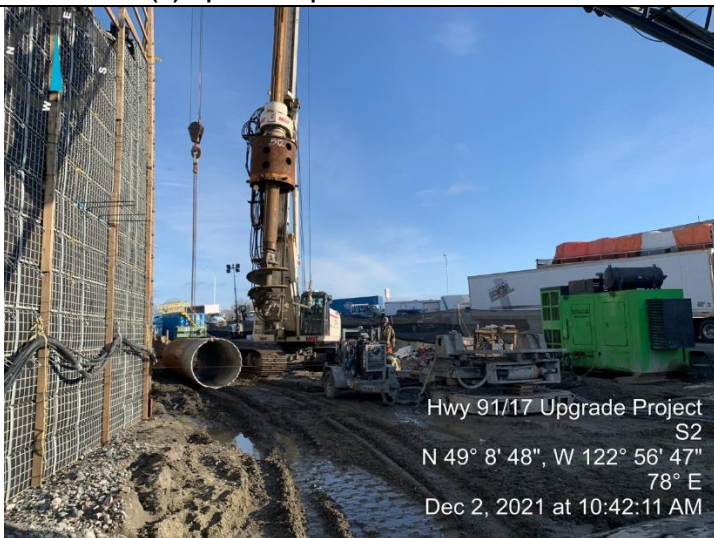
Photo 3: L500 (E). Drill shaft installation on S2 bridge.
