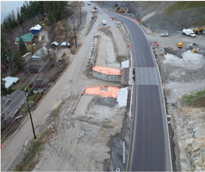
Progress on the Old Sicamous Road Overpass (December 2025)
