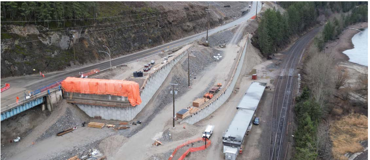
R.W. Bruhn Bridge west abutment progress (December 2025)
