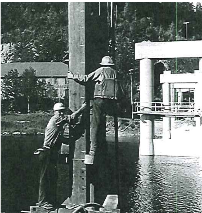
Pile driving for Pier #4 on the original R.W. Bruhn Bridge (June 1962)
