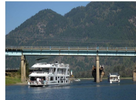
Trans-Canada Highway 1 RW Bruhn Bridge and Approaches Project
