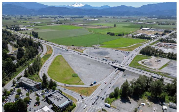
Construction started this spring on the Highway 11 Interchange Project.
