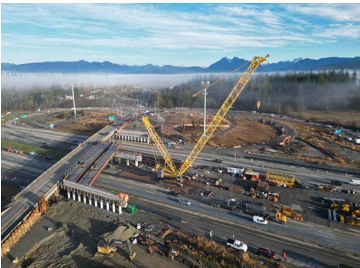
Girder installation at the 232nd Street Interchange.
