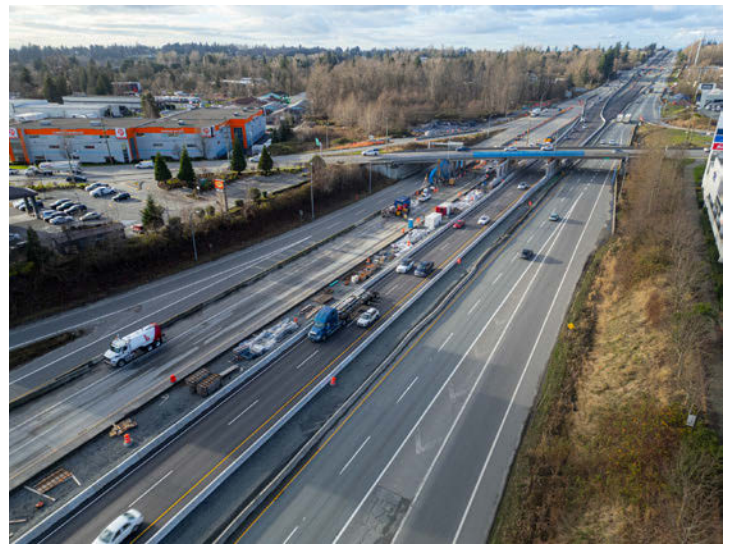
Lane shifts as part of the Mt Lehman Interchange Project.
