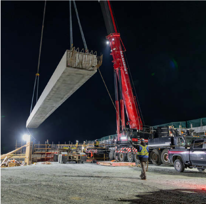
Girder installation at Bradner Road.
