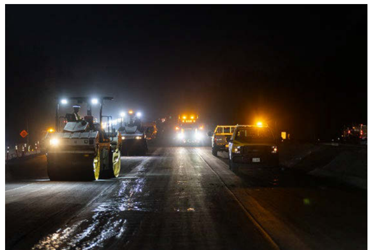
Nighttime paving operations in preparation for highway widening.
