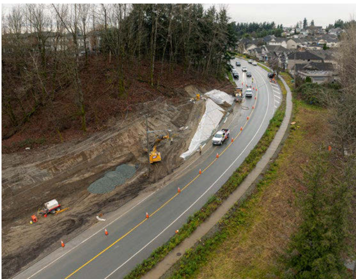
King Road realignment work to make room for the Highway 1 expansion.
