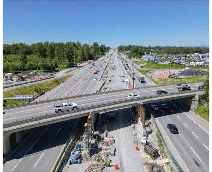
Preparation for lane widening happens at the Mt. Lehman underpass.
