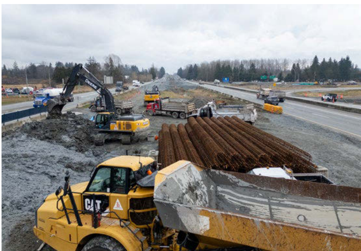
Workers prepare for pile installation at the 232nd street interchange.
