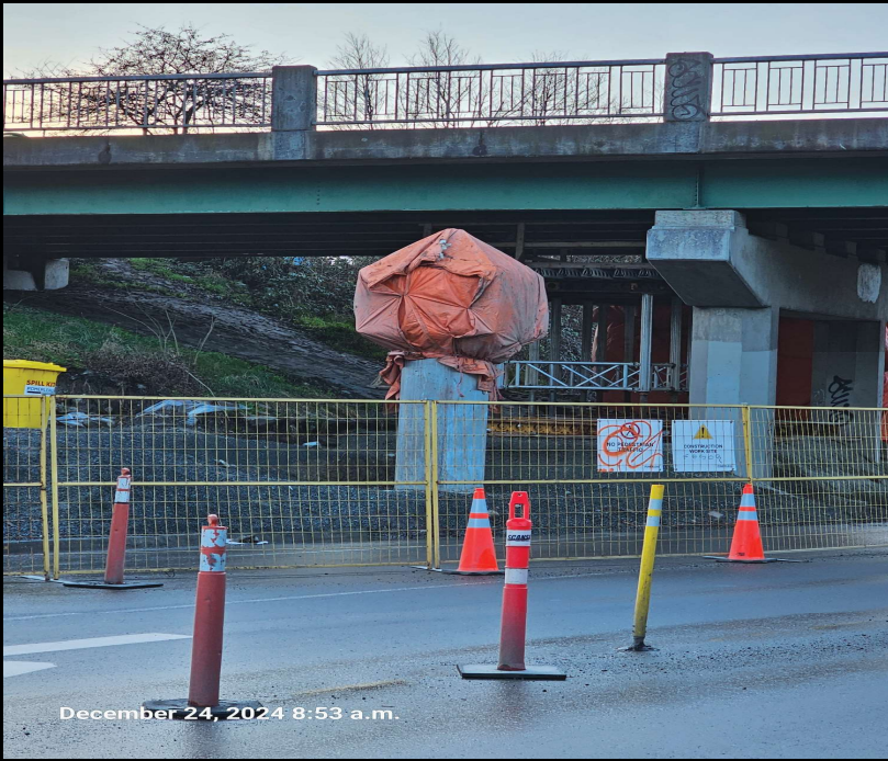
Figure 2: Installation of New Bent at the North Bridge
