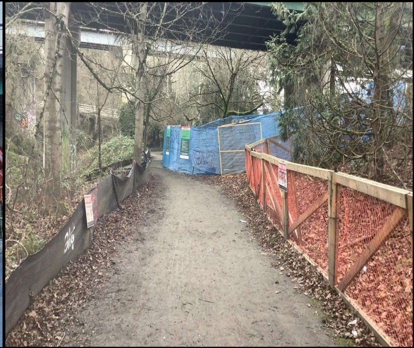
Figure 3: Ongoing Maintenance of Snow Fencing and Tree Protection Fencing
