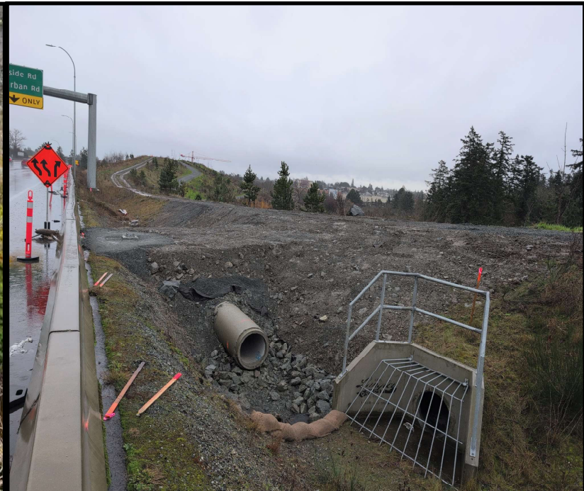
Figure 5: Completion of New Culvert
