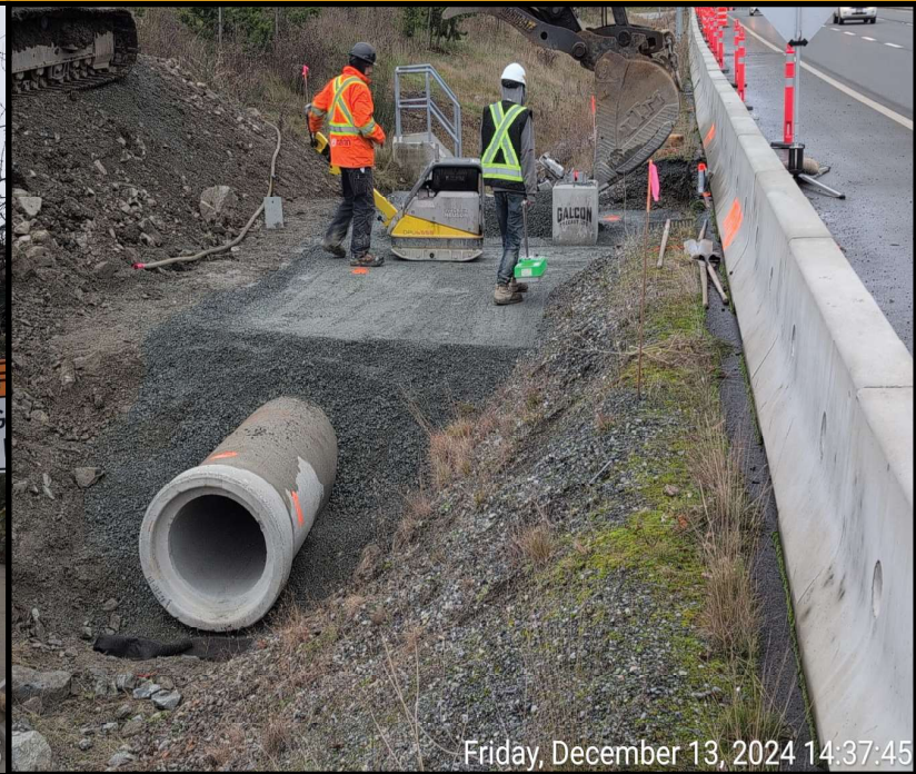
Figure 3: Highway 1 Culvert Installation
