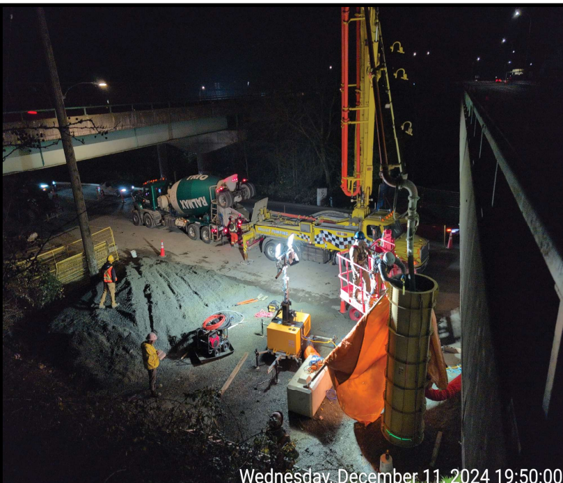
Figure 4: North Bridge Pile Installation
