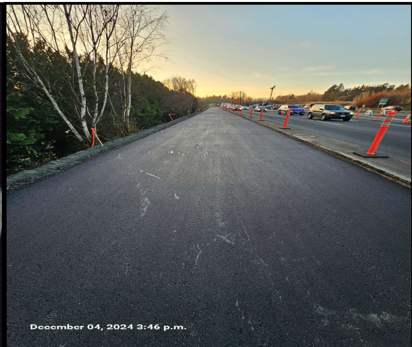
Figure 5: Highway 1 Paving Works
