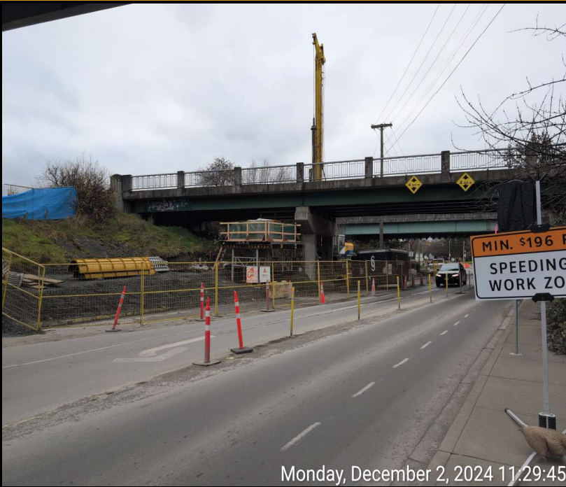
Figure 2: Works Along North Bridge
