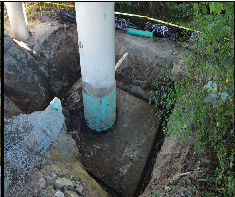
Figure 5: South Bridge Existing Pier Work
