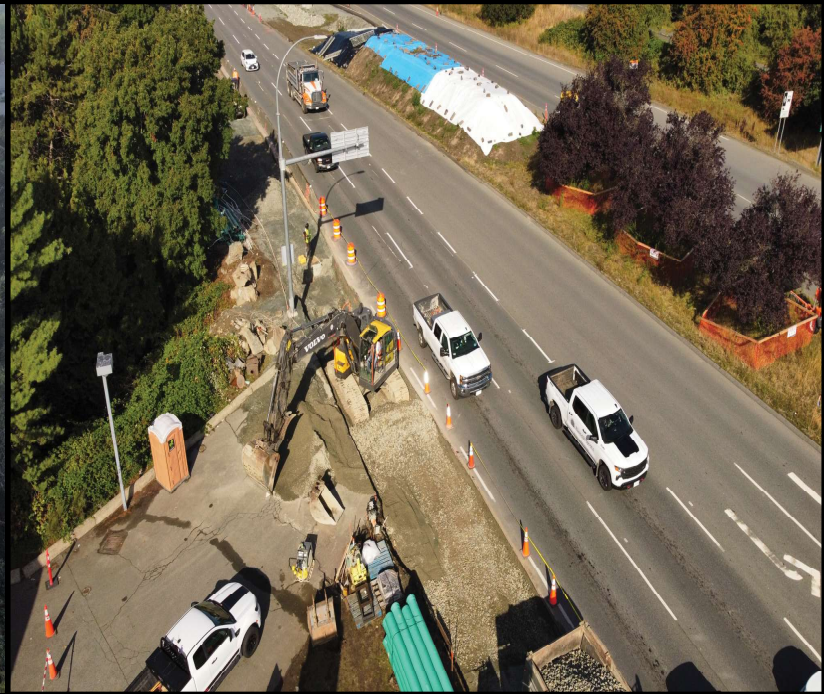
Figure 3: Roadworks Along Highway 1
