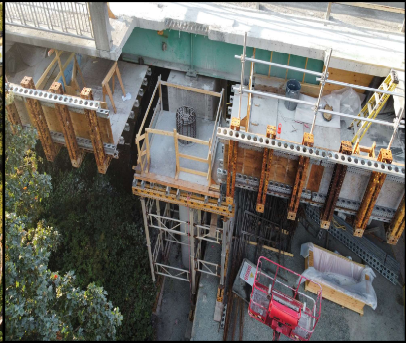
Figure 3: Pile Installation at South Bridge
