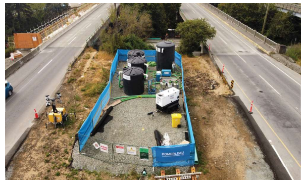
Figure 1: Water Treatment Facility
