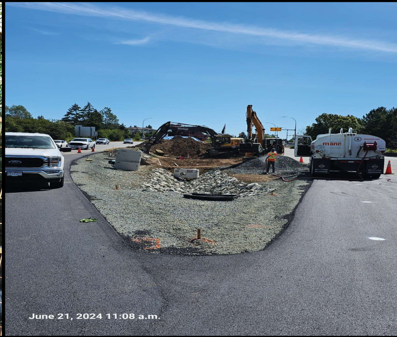
Figure 3: Paving of the Temporary Median Crossover
