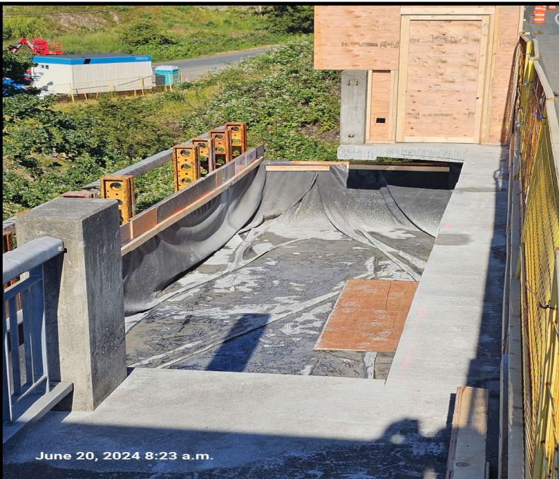
Figure 4: South Bridge Slurry Containment
