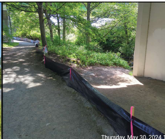
Figure 2: Silt Fence Established to Prevent Mitigation of Sediments into the Colquitz River
