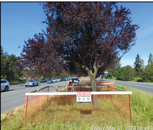
Figure 1: Tree Protection Fencing Around Trees in the Median
