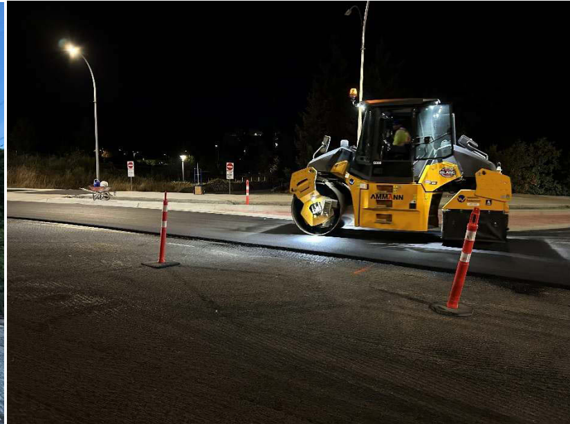
Paving installation at Helmcken Interchange
