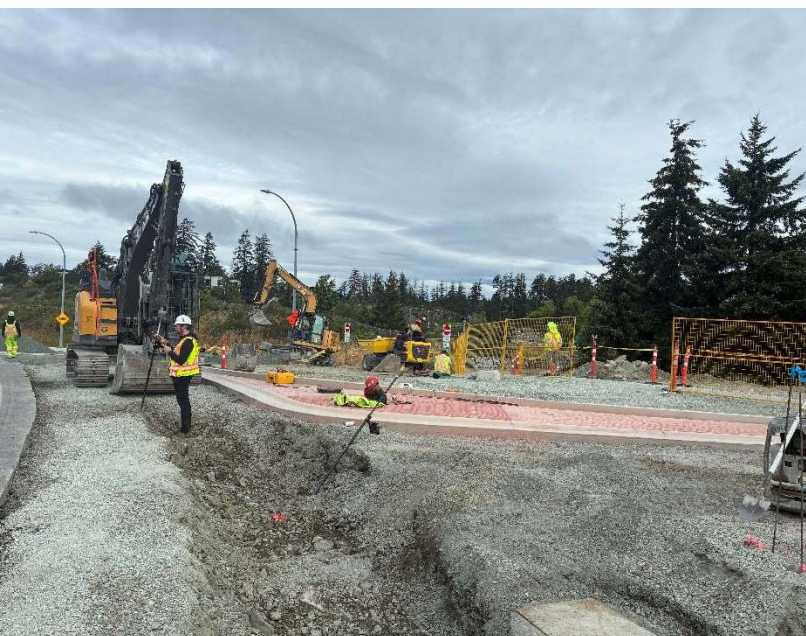
Helmcken Interchange new island construction
