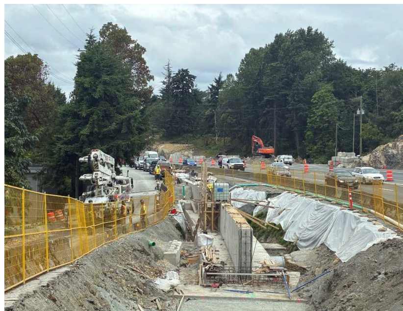
Portage Road retaining wall construction
