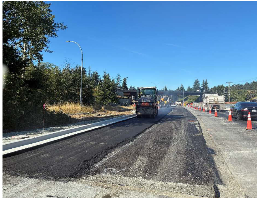
Paving works on Burnside Rd West
