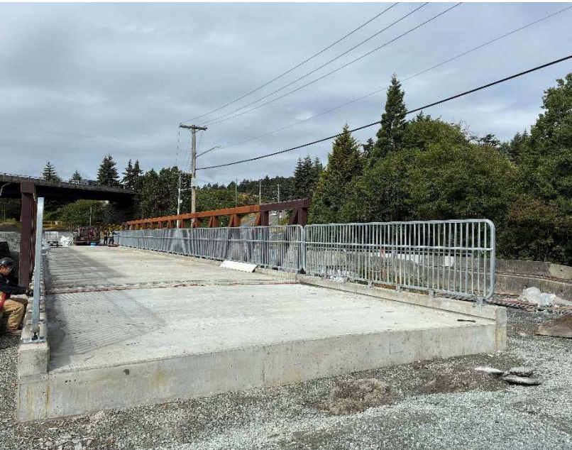
Galloping Goose Trail multi-use bridge construction
