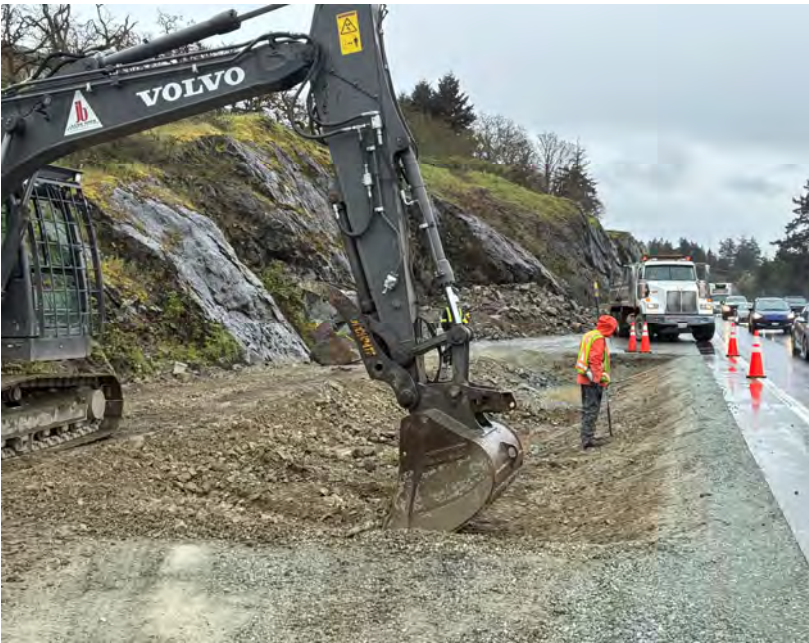
Grading works along Highway 1, east of Wilkinson pump station
