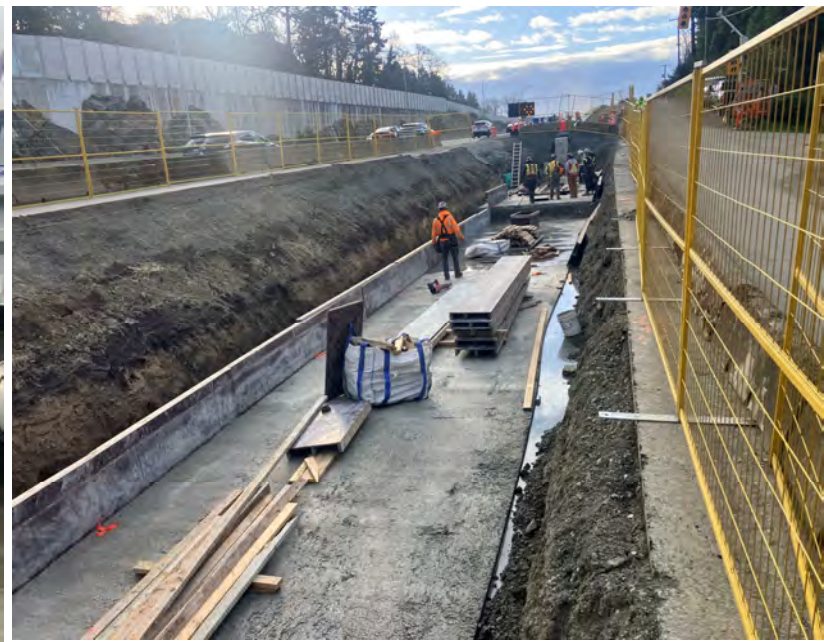
Portage Road retaining wall construction
