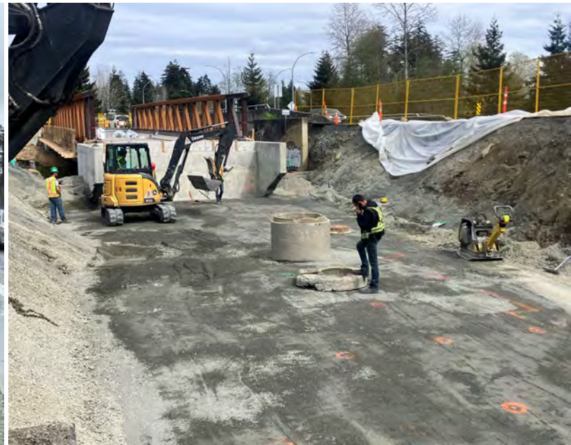
Galloping Goose Trail multi-use bridge construction
