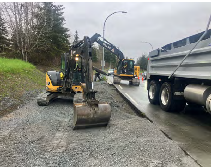
Road widening works at Burnside Rd West (Highway 1 offramp to Colwood)
