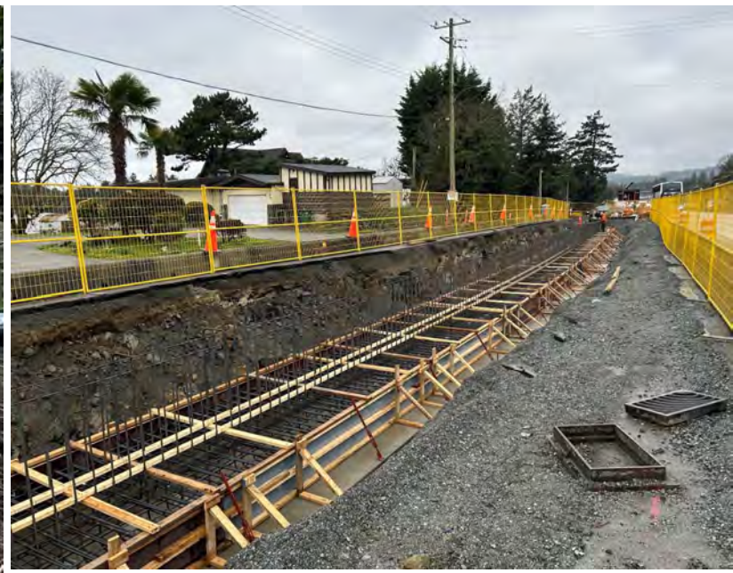
Portage Road retaining wall construction
