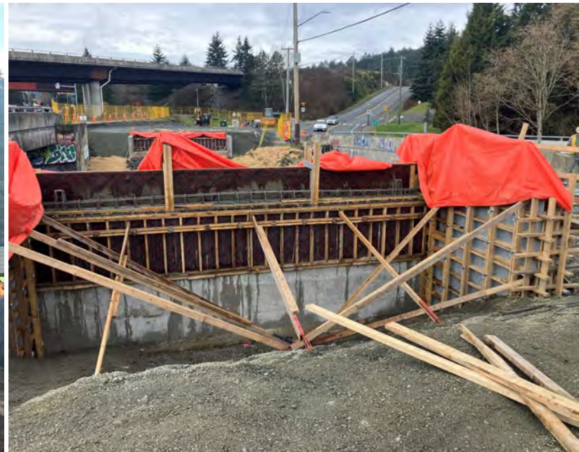
Galloping Goose Trail multi-use bridge abutment construction
