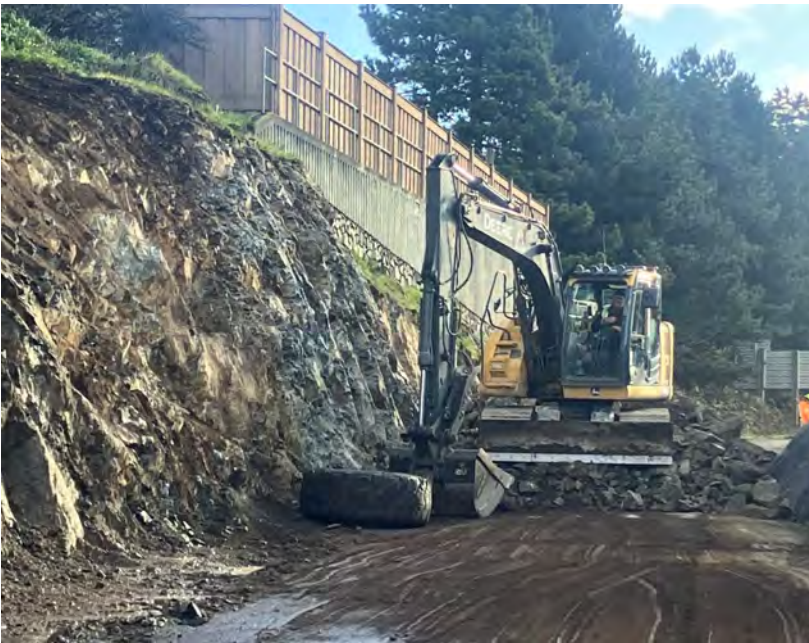
Rock removal along Highway 1, east of Wilkinson pump station
