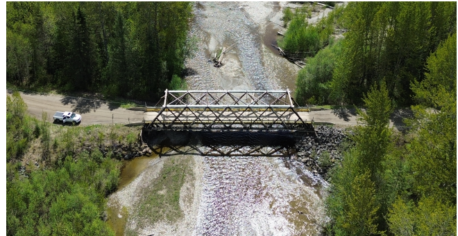
Drilling will be conducted near Ahbau Creek Bridge.
