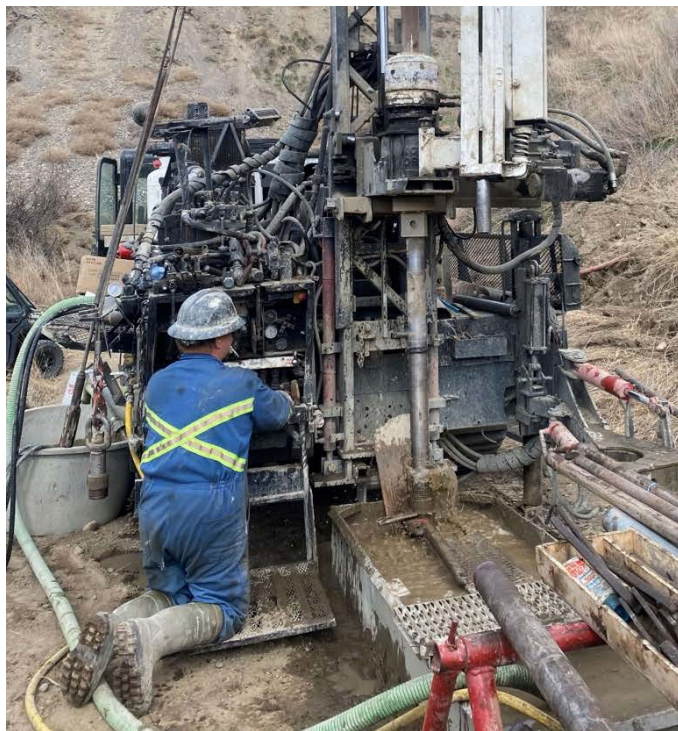
Example of geotechnical drilling equipment.
