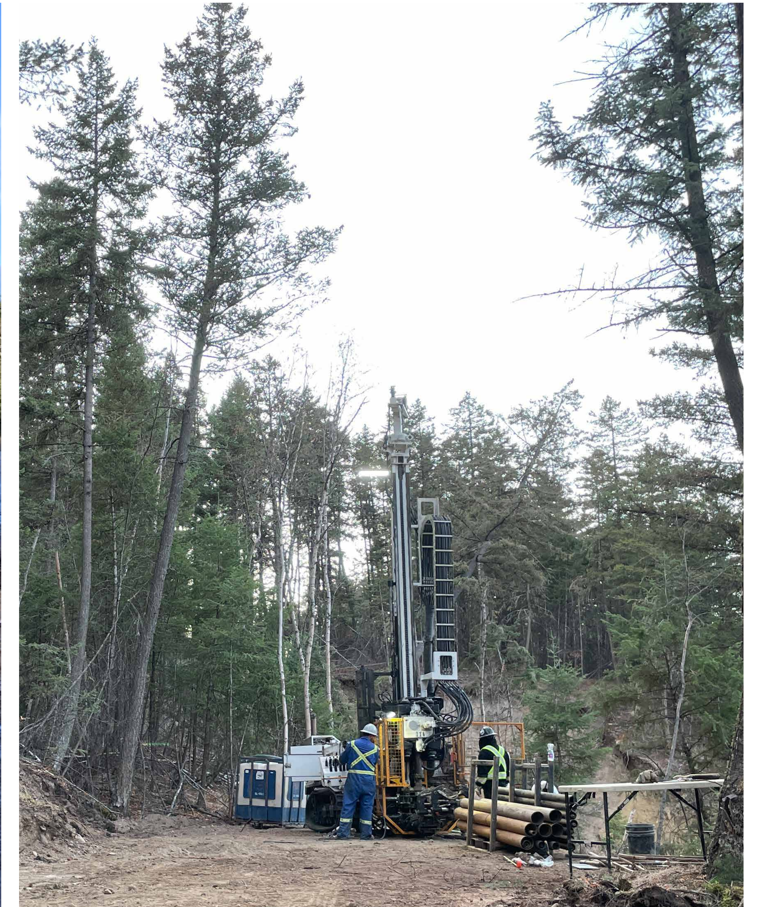
Geotechnical drilling was completed last fall near the Dog Creek Slide.
