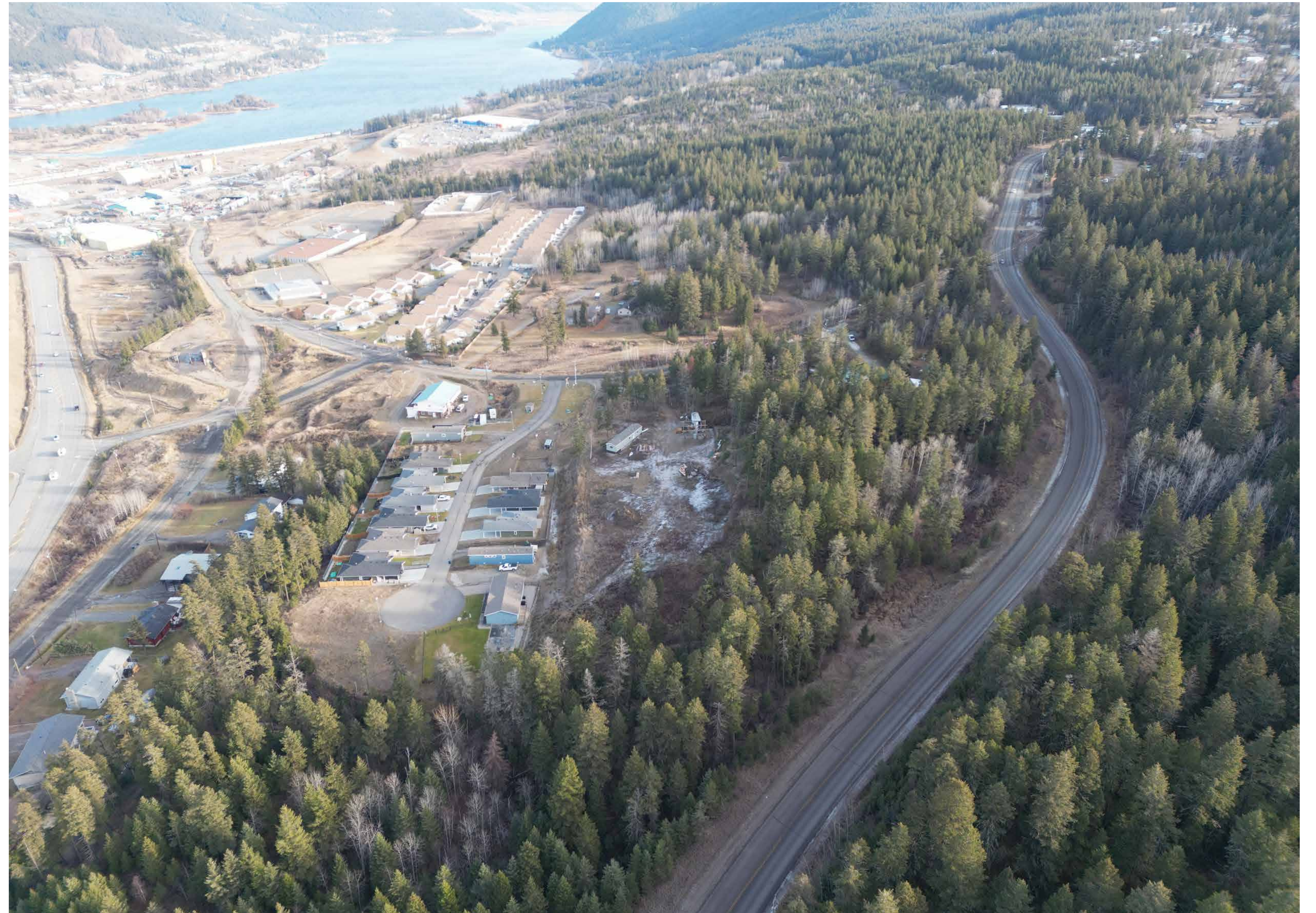
Aerial image of the project area, looking east, with Dog Creek Road on the right and Highway 20 on the left. Most of the Hodgson Slide is located in the City of Williams Lake. The Dog Creek Slide is split between City and Cariboo Regional District jurisdiction.
