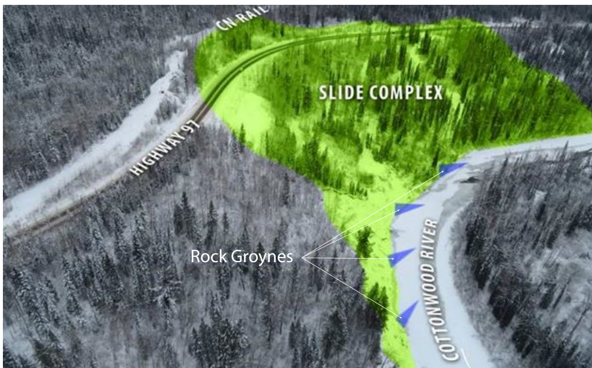
The location of the four groynes installed in the river this fall.
