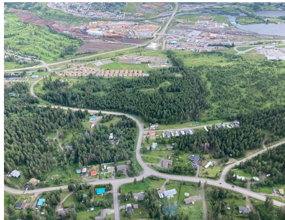
Aerial view of the Hodgson Slide area, looking north toward downtown Williams Lake.
