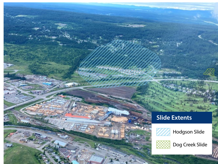
The area of this project includes the Hodgson Slide and Dog Creek Slide.
