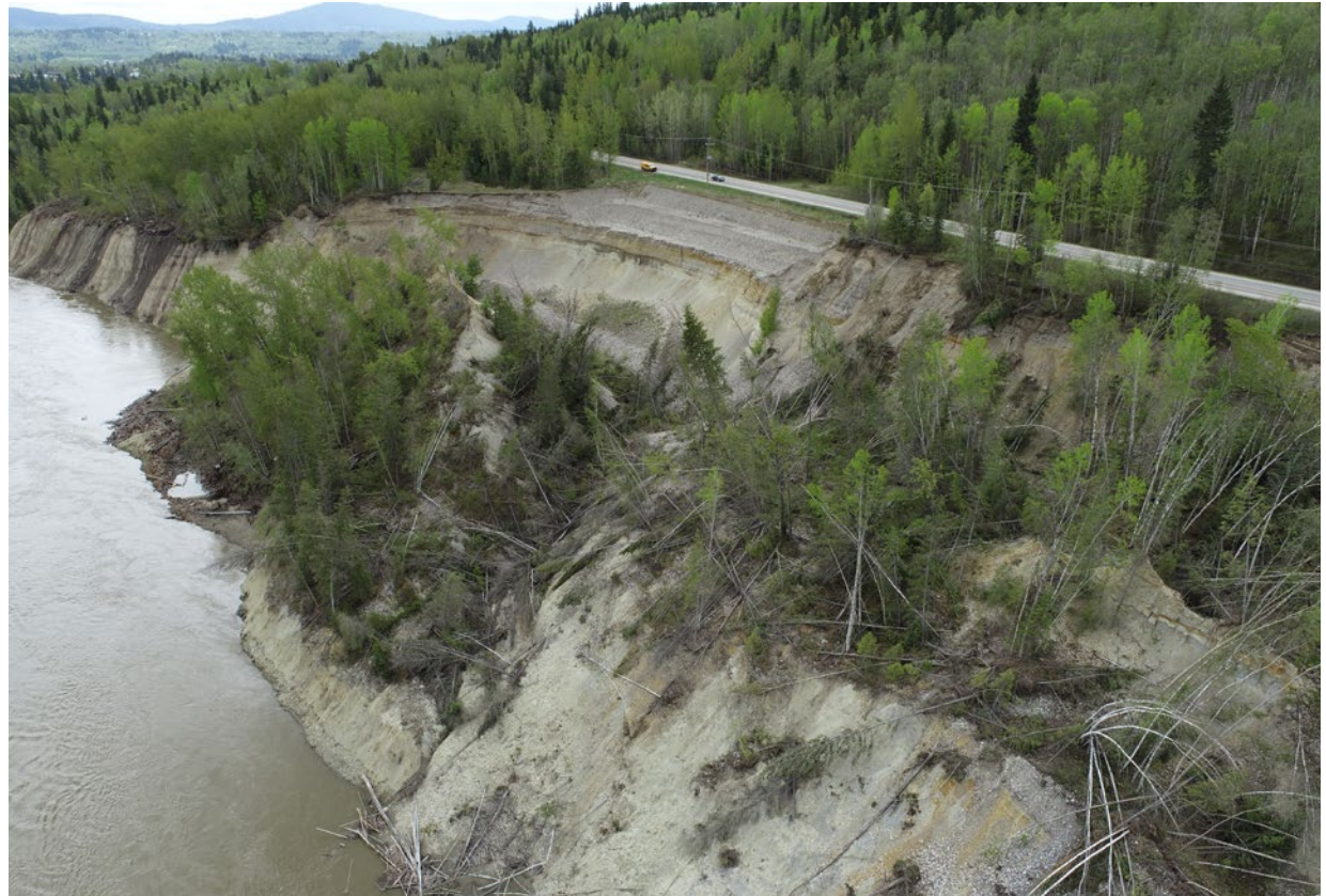
Photo of the embankment to be stabilized along the Fraser River.
