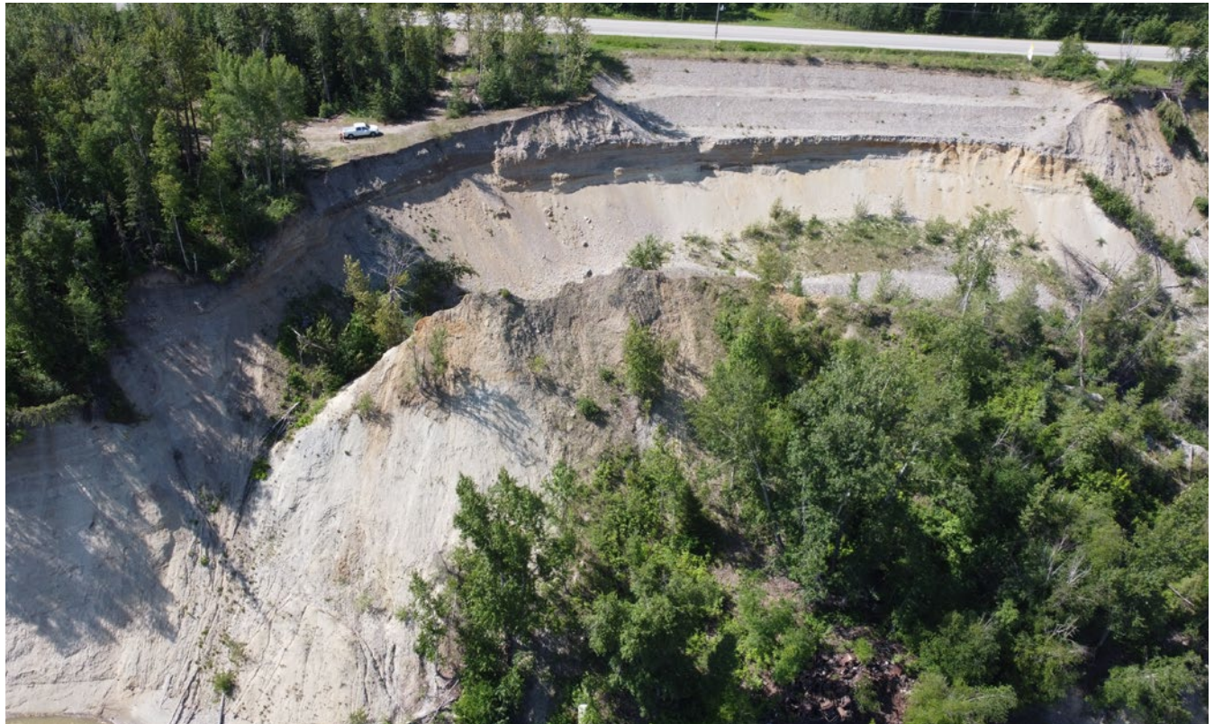
A view of the North Fraser slide from above the Fraser River.
