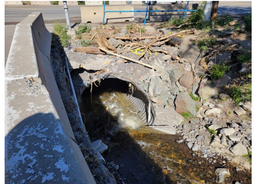
The culvert that runs under Highway 97. Photo taken in June 2023.
