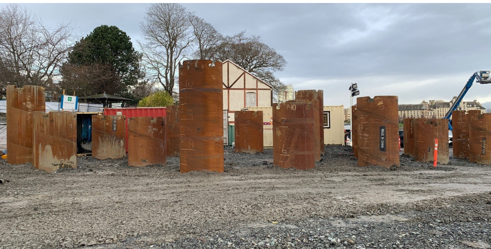
View of temporary pile casings beginning to go in on site.
