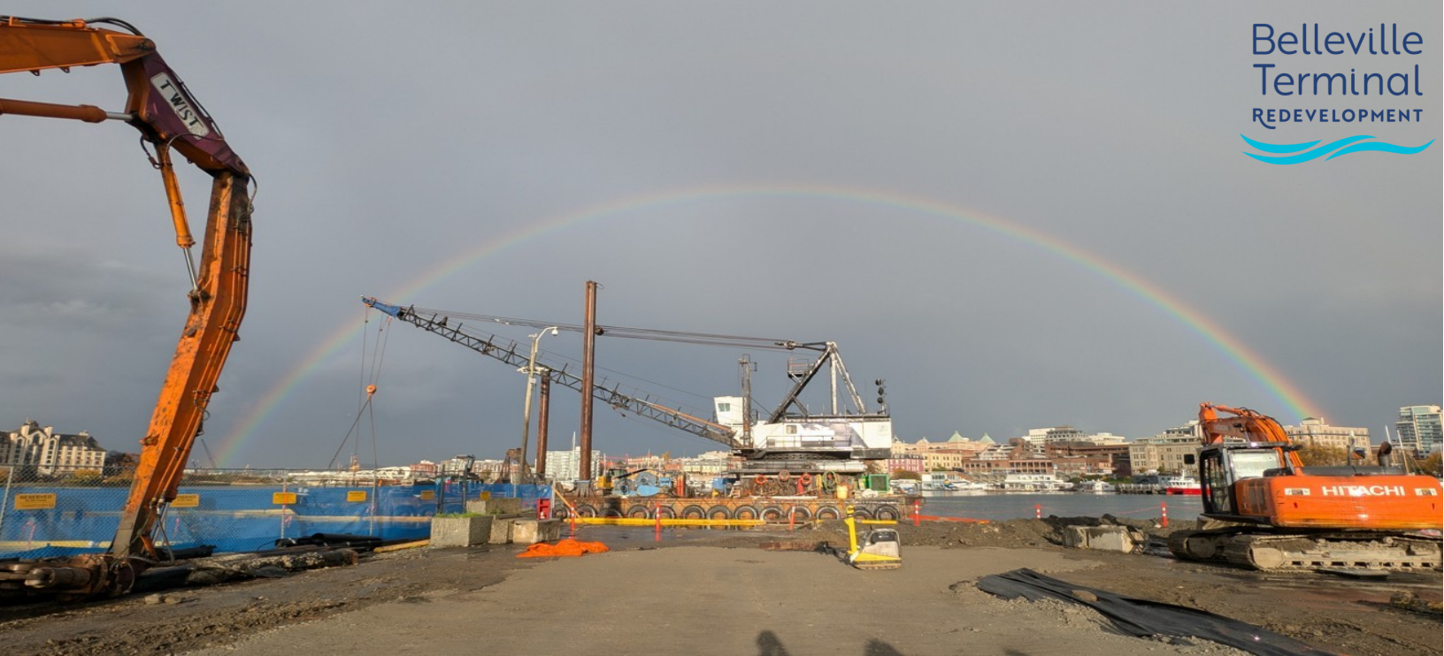
View of barge crane.
