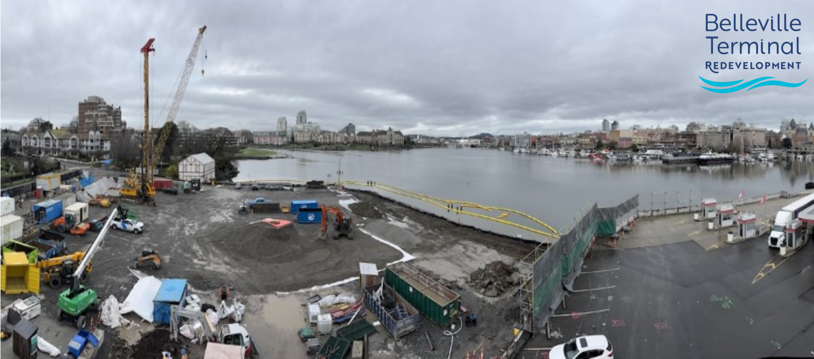
View of construction site.
