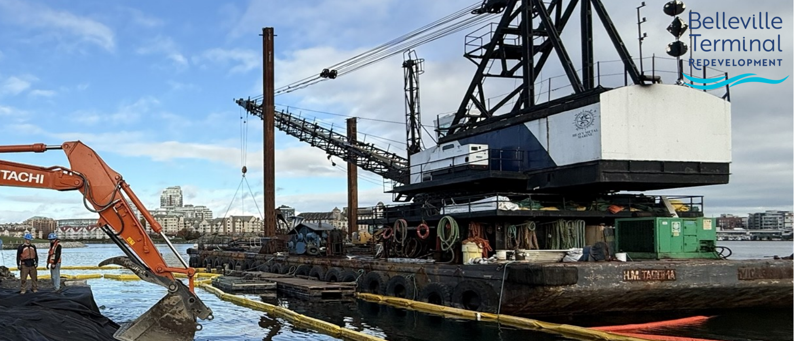
View of site machinery and workers.
