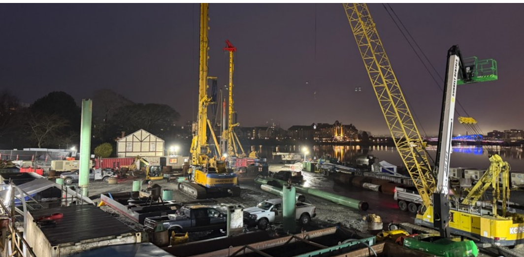
View of site machinery.
