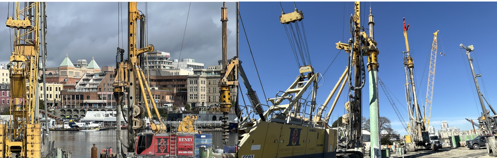
View of site machinery.
