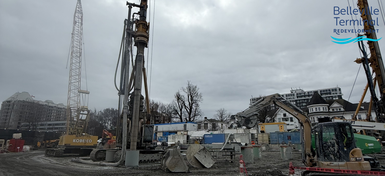
View of site machinery looking south.
