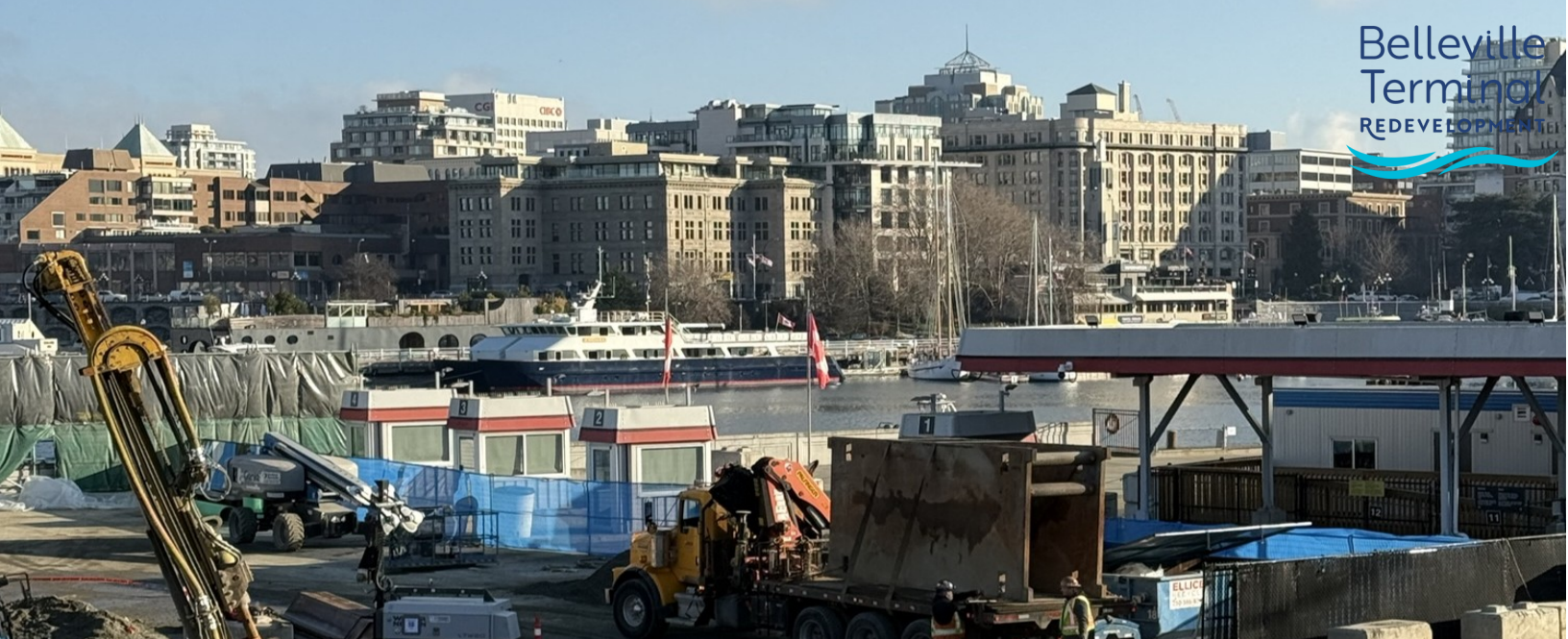
View of site machinery.
