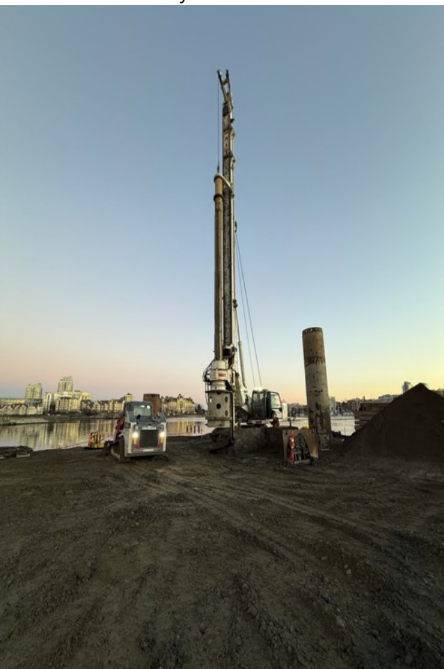
View of site machinery.
