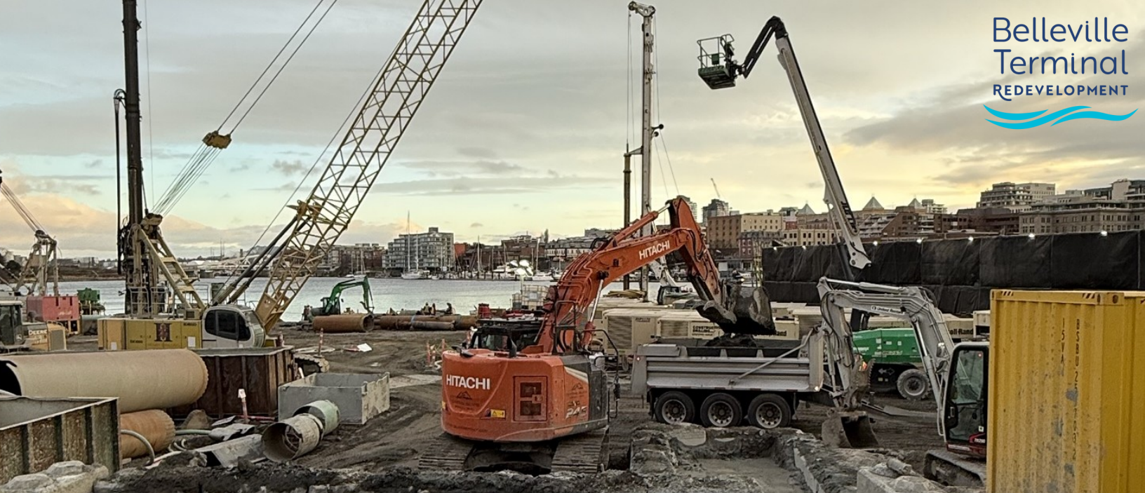
View of site machinery.
