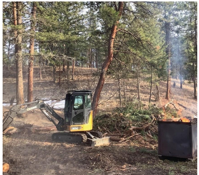
Figure 18. Burn box for debris management to limit site disturbance during a fuel management project in Ellison Provincial Park.
