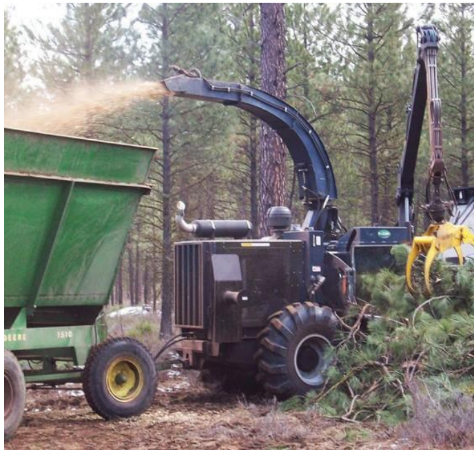
Figure 26. Implementation of cut, chip, and haul for debris management.
