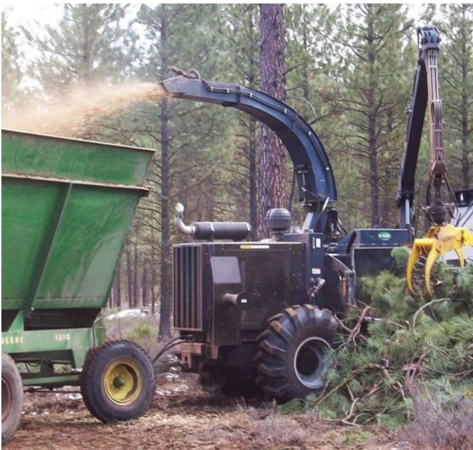
Figure 33. Implementation of cut, chip, and haul for debris management.
