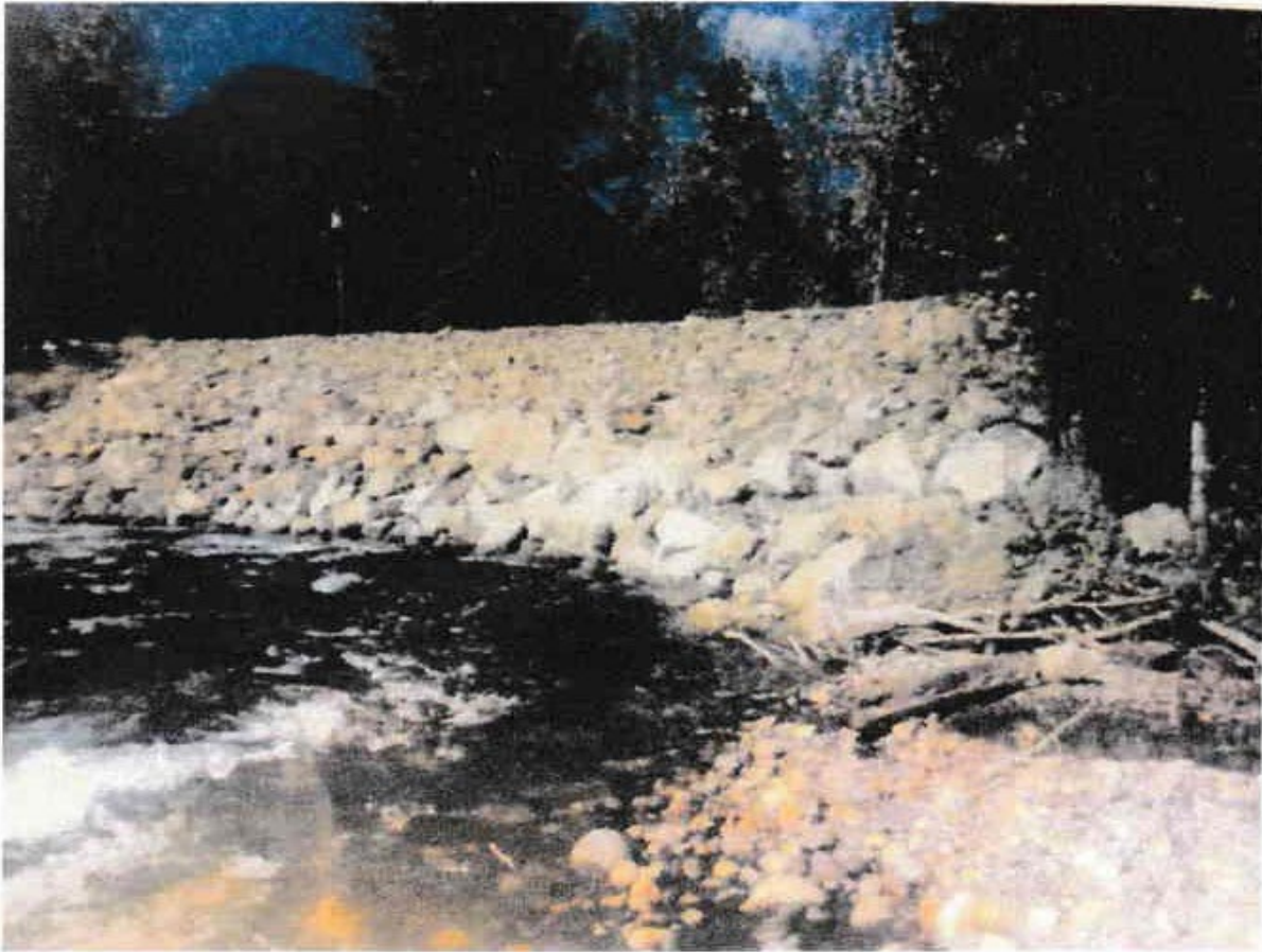
Figure 11: Site 5 View of repaired dike photo from September 2014 (CGT 2014)
