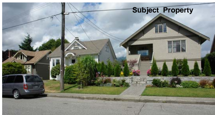
Street view of front unit (on right side of photo) and adjacent single family dwellings
