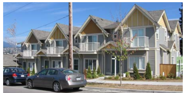
Street view of the units from Gilmore Avenue
