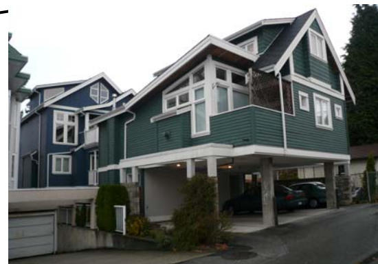
View from lane: coach house over open carport. Note different, but complementary colours for main structure and coach house.
