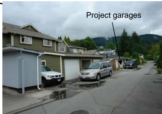
View of rear lane
