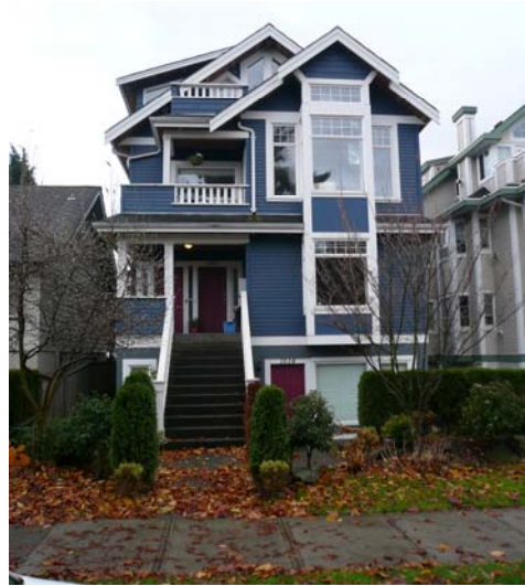
Careful placement of entry doors to three units contributes to single detached look.
