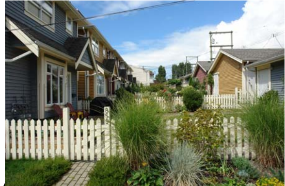
View from Campbell Avenue showing fencing, landscaping detail, and yard between rear unit and garage
