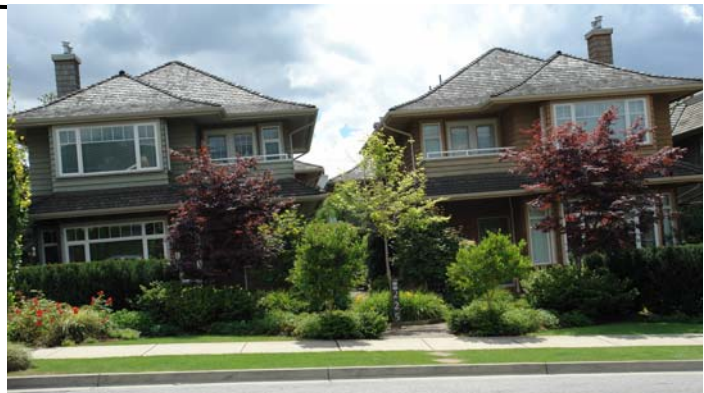
Street view of the two front units
