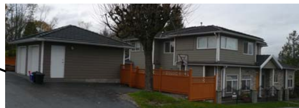
View of the shared garage from Gilmore Avenue
