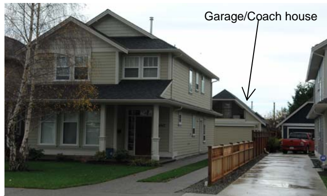
Street view of one of the single family units with a view through to the garage/coach house in the background
