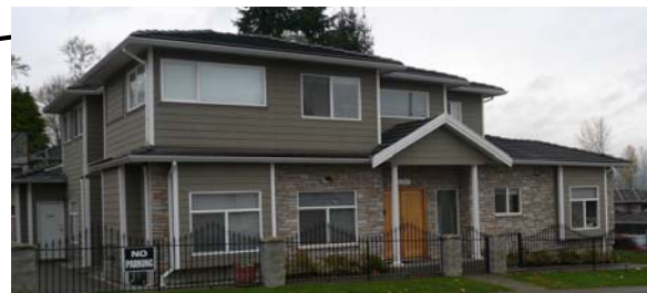
Street view of the unit facing Gilmore Avenue (3109 Gilmore)
