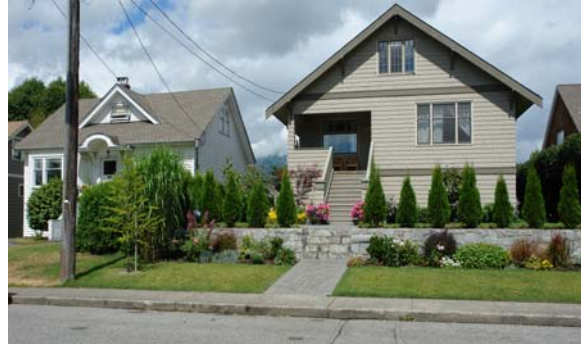
View of older, renovated house.
