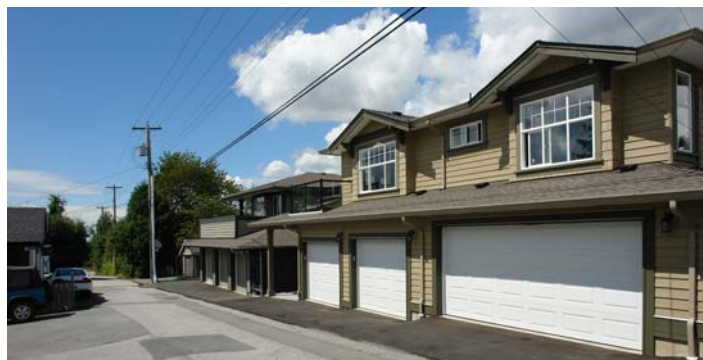
Lane view showing garage with unit above
