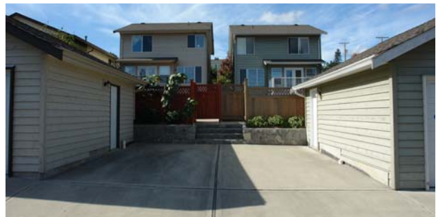
View of the project garages, parking pad, and rear of the units
