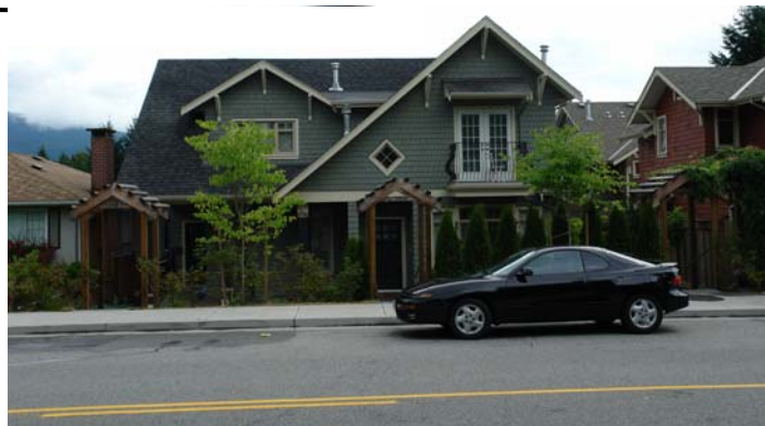
View from Fromme Road. Note three trellis gates marking entry paths to the individual units
