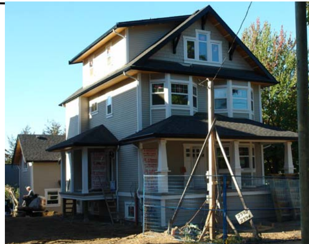
View showing entrances on north and east sides
