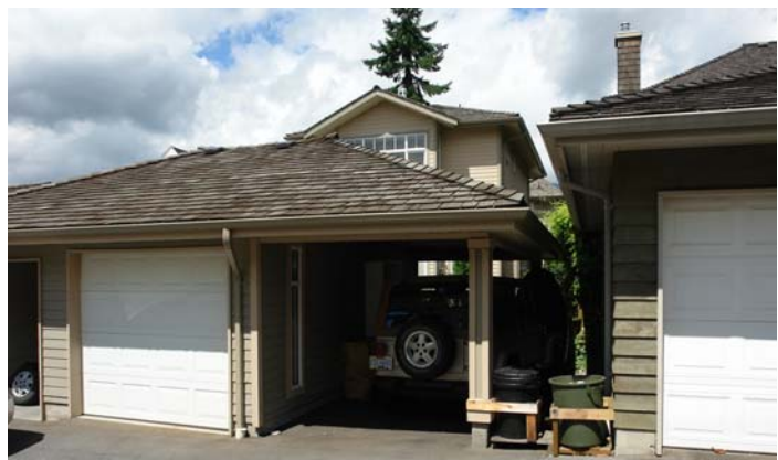
Lane view of the garages and rear units
