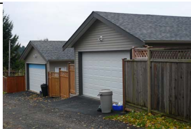
View of the project's garages, which are accessed off the rear lane
