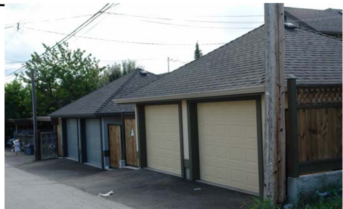
Lane view of the garages
