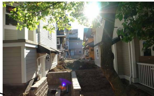
View of separation between main structure and coach house/garage structure
