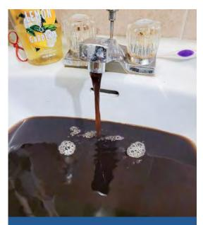
A customer supplied by the Town of Osoyoos water system experienced a slug of manganese deposits in their drinking water after a nearby hydrant was disturbed. Physical disturbances to a distribution system can cause the release of manganese deposits from pipes. In June 2023, the Town of Osoyoos was granted \$9 million to assist with water infrastructure projects to improve drinking water quality. *Photo credit: Jessica Kriese, Osoyoos, BC.*
