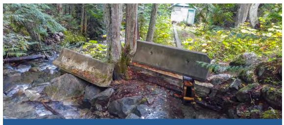
Sandy Creek Water Users' Community near Nelson, BC. The intake of Sandy Creek leads to a concrete reservoir. The system supplies 83 connections via gravity but has no treatment, and a long-term boil water notice has remained in place for more than three decades. *Photo credit: Greg Baytalan, Environmental Public Health, Interior Health.*
