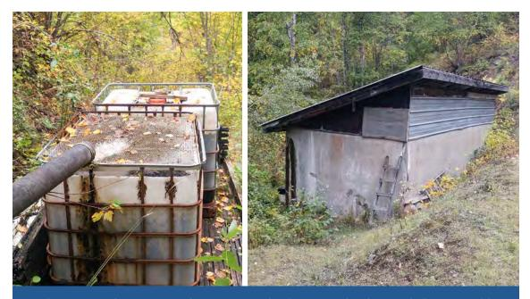
A small water system in the West Kootenays of BC's interior. Diverted creek water passes through a screened collection system (left) to remove sticks, leaves, and debris before entering the storage reservoir (right). Water is delivered to homes on the system by gravity with no further treatment. The water system has been on a boil water notice for more than 30 years. Untreated drinking water is the most common cited reason for drinking water advisories in BC.
