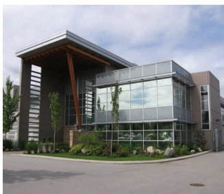
Fraser Health's Support Services Facility located in Langley, BC.
