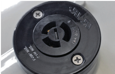
NEMA 3-pin rotatable receptacle
