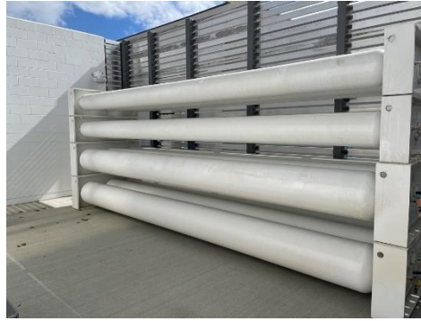
Figure 6: Example of ground storage tank
