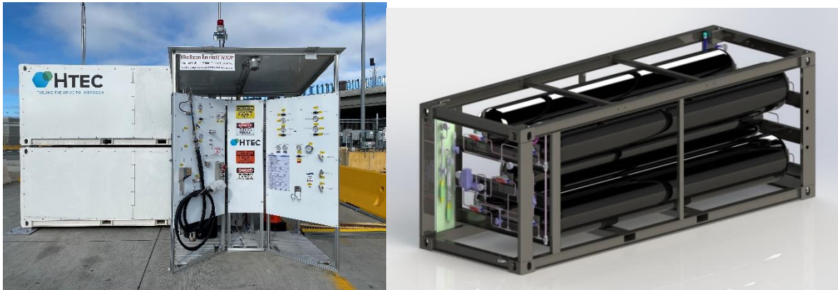
Figure 9: 4 HTEC PowerCubes stacked for on-site storage at the Port of LA (left) 19 , view of single HTEC PowerCube (right)
