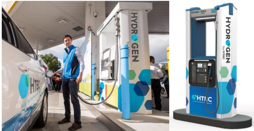
Figure 7: Light-Duty Station Refuelling; Hydrogen Dispenser
