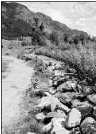
Rip rap to prevent bank erosion.
