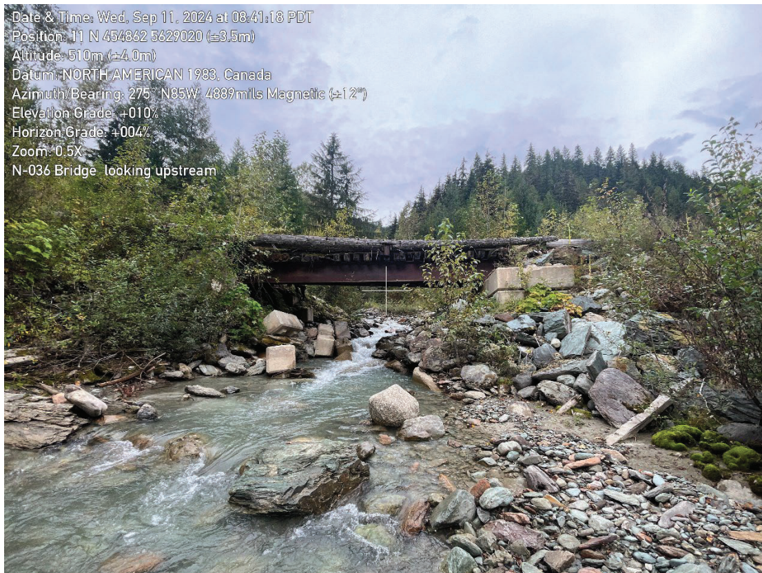
Overview of N5-036 bridge looking upstream.
