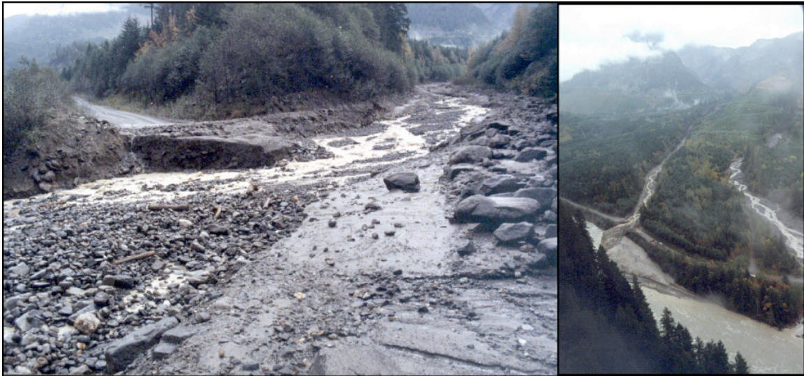
Figure 3. Washout at Turbid Creek in 1997. Exact date of occurrence unknown (from photos on file with Friele). Note this is a typical small, channelised event; it destroyed the crossing and filled Squamish River with debris, and may have briefly dammed the river.
