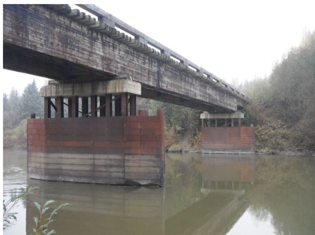
Bridge Site G1-115
