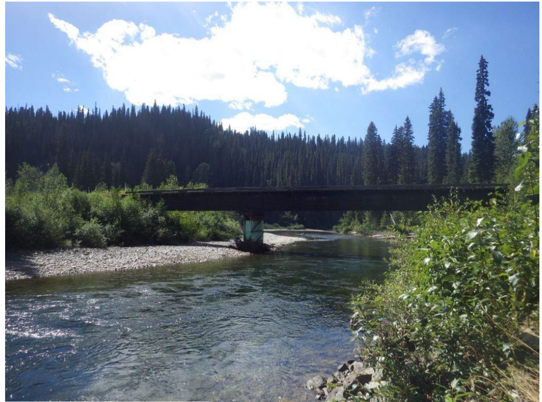
Bridge Site G1-046
