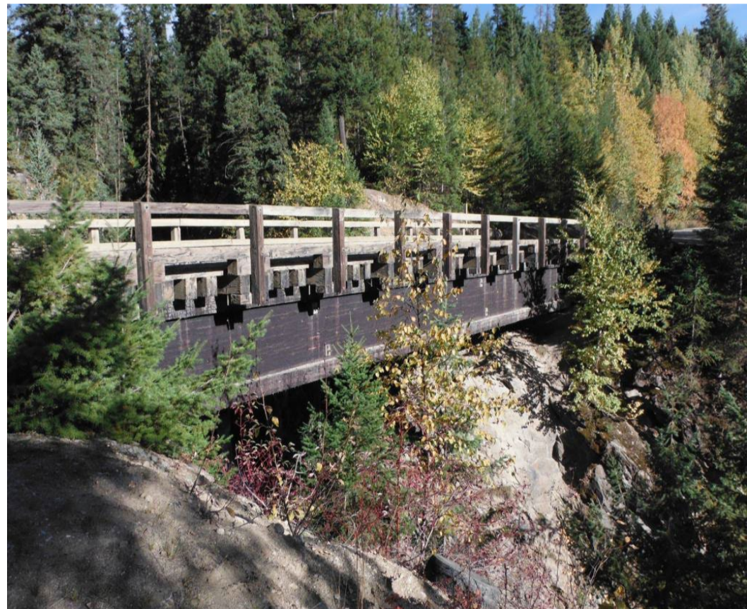
Bridge Site G3-012
