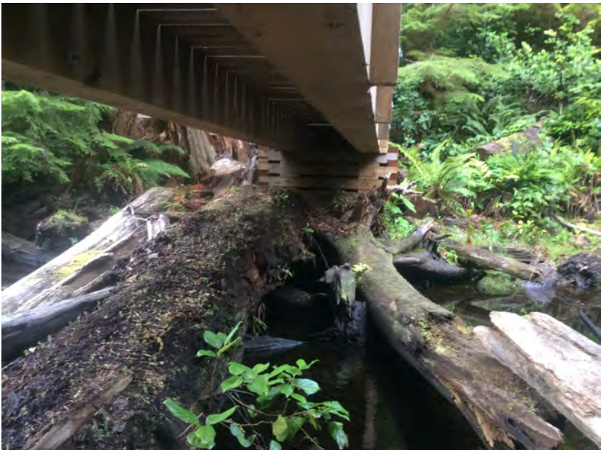
Left Bank Abutment when facing downstream
