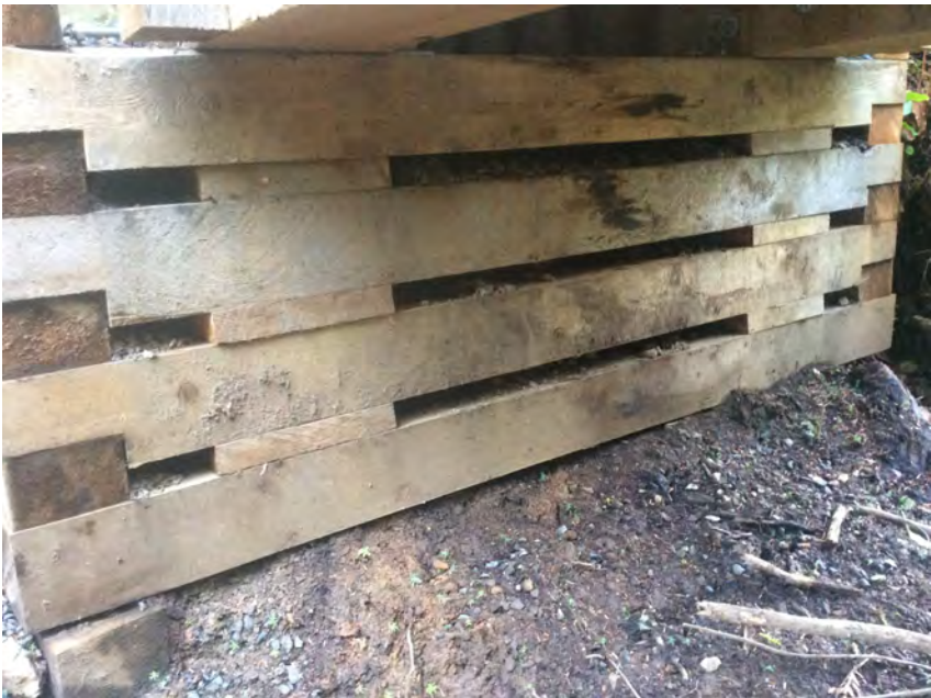
Right Bank Abutment when facing downstream
