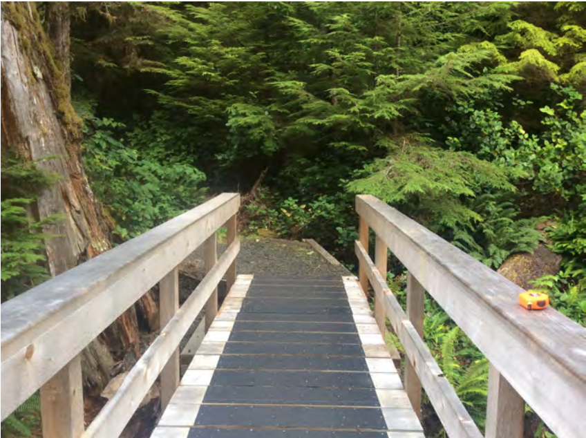
Centre of bridge to river left approach
