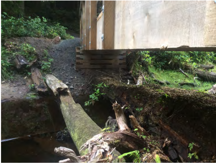
Right Bank Abutment when facing downstream
