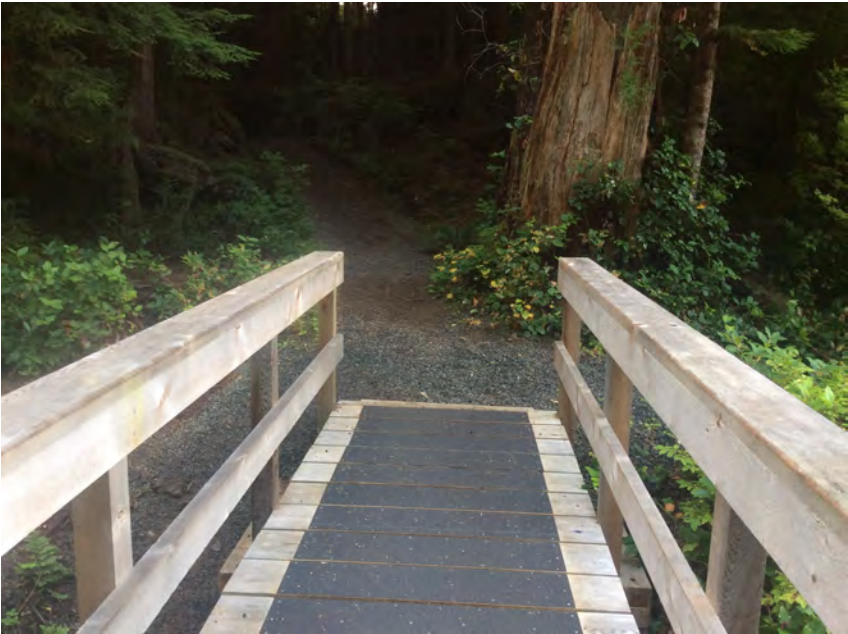
Centre of bridge to river right approach
