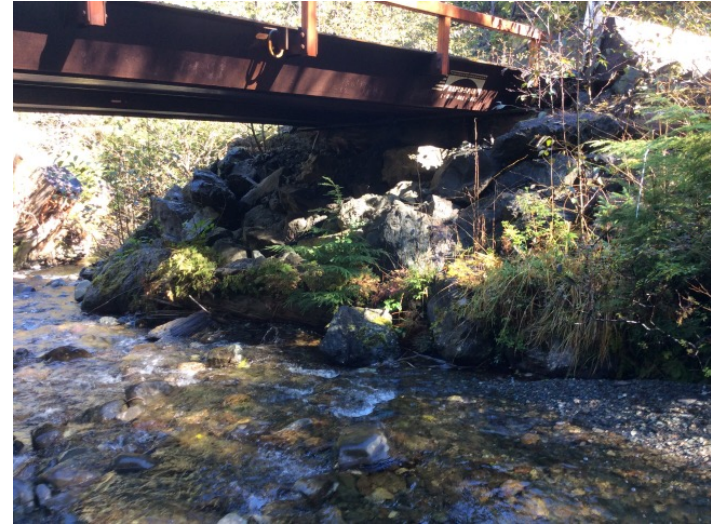
Right Bank Abutment when facing downstream
