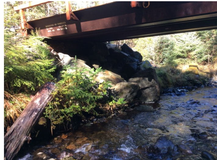
Left Bank Abutment when facing downstream
