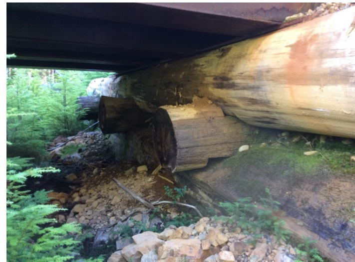
Left Bank Abutment when facing downstream
